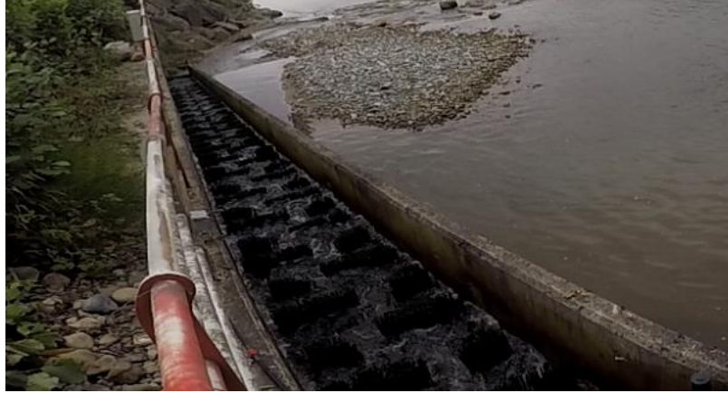
Figure 1.4 : View from the field: Brush based fishway model setup on small hydropower plant in İkizdere River, Rize, Turkey is used in experiments.
