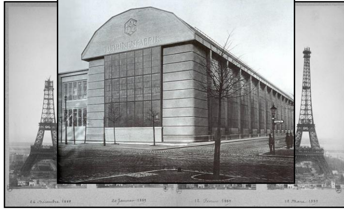
Şekil 5.2. Eiffel Kulesi, Fransa,1889 ( https://rarehistoricalphotos.com/eiffel-tower-construction/ )
