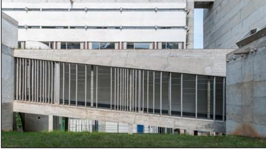
Şekil 6.30. Ritmik cepheye sahip beton koridor ( https://www.archdaily.com/96824/ad-classics-convent-of-la-tourette-le-corbuiser )
