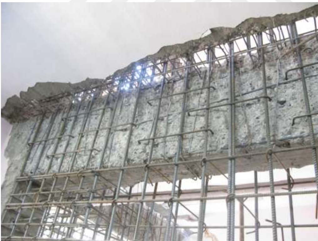
Figure 1.3 : Anchors functioning as cross-ties.
