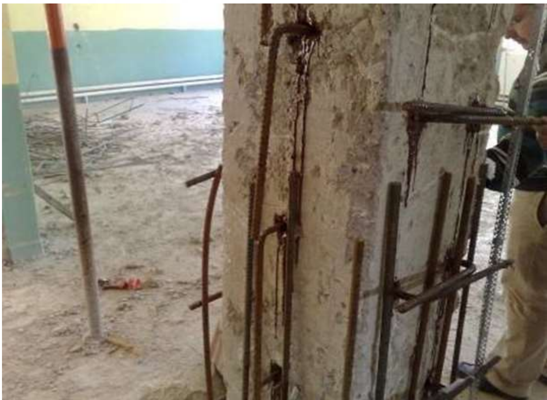
Figure 1.1 : Anchors in jacketing of column [4].
