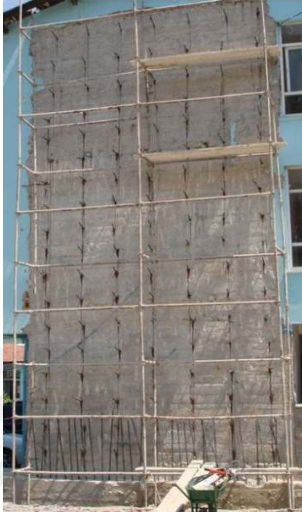
Figure 1.4 : Anchors in external shear wall application [4].
