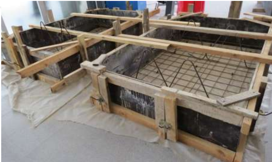
Figure 3.6 : Mold prepared for pouring of concrete
