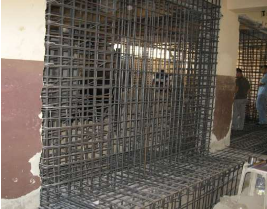
Figure 1.2 : Anchors connecting infill shear wall to frame.
