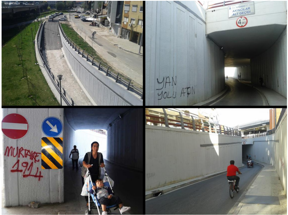
Figure 5.22: Underpass which connect the neighborhood to city center
