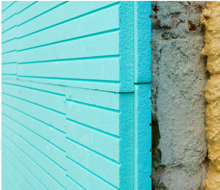
Figure 3.12 : Wall being insulated with XPS panels.
