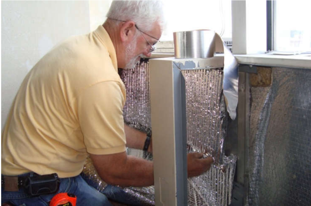
Figure 3.39 : GFP being applied for insulation.
