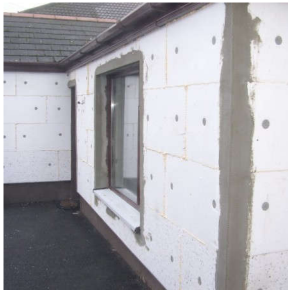
Figure 3.10 : Wall being insulated with EPS panels.
