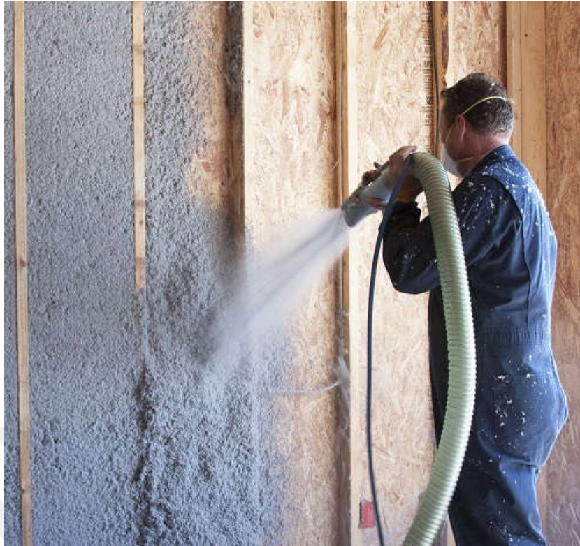
Figure 3.44 : A wall being insulated with cellulose.
