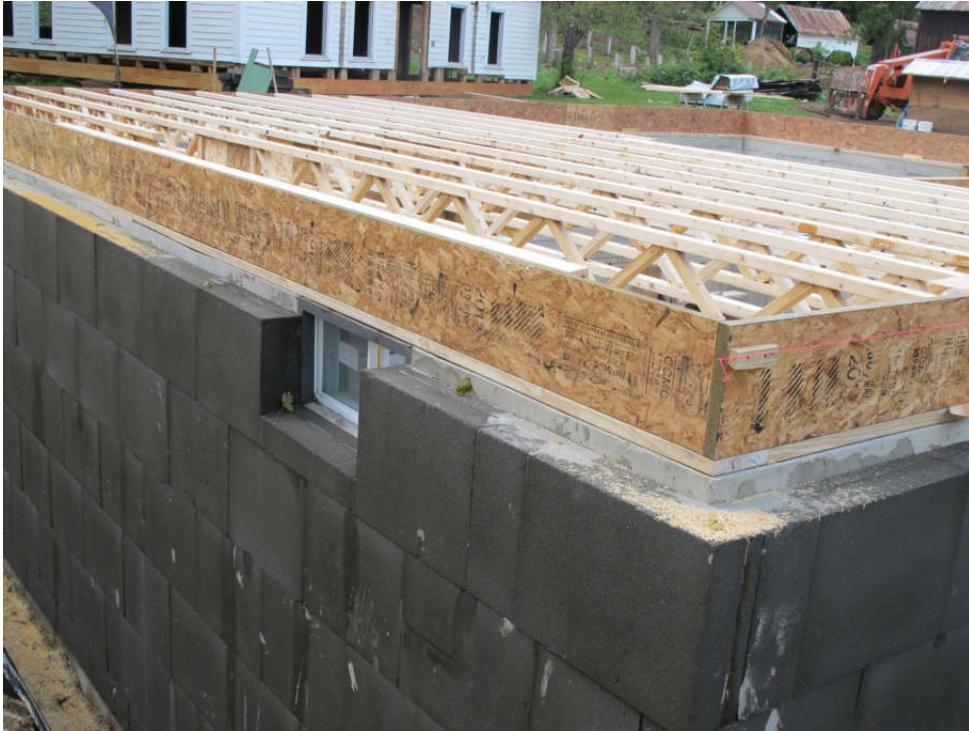
Figure 3.8 : Basement floor walls insulated with foam glass.
