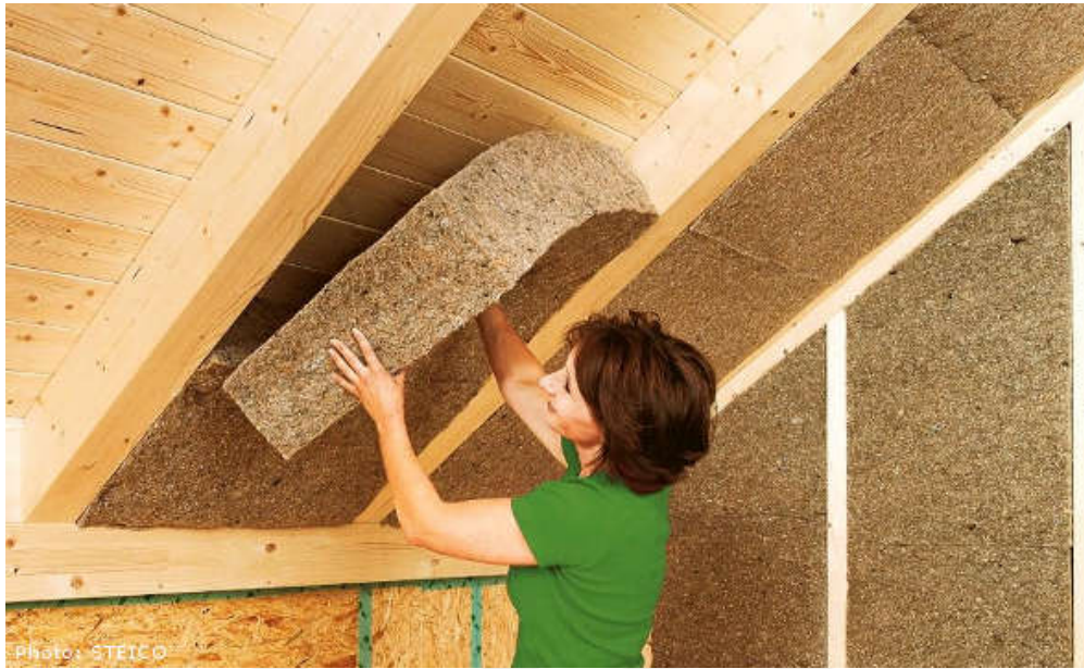
Figure 3.17 : Roof being insulated with hemp panels.
