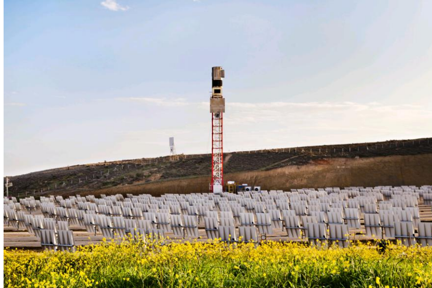
Figure 4.8 : Mersin project, Turkey [20].
