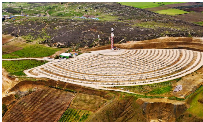
Figure 4.9 : Mersin project, Turkey [20].
