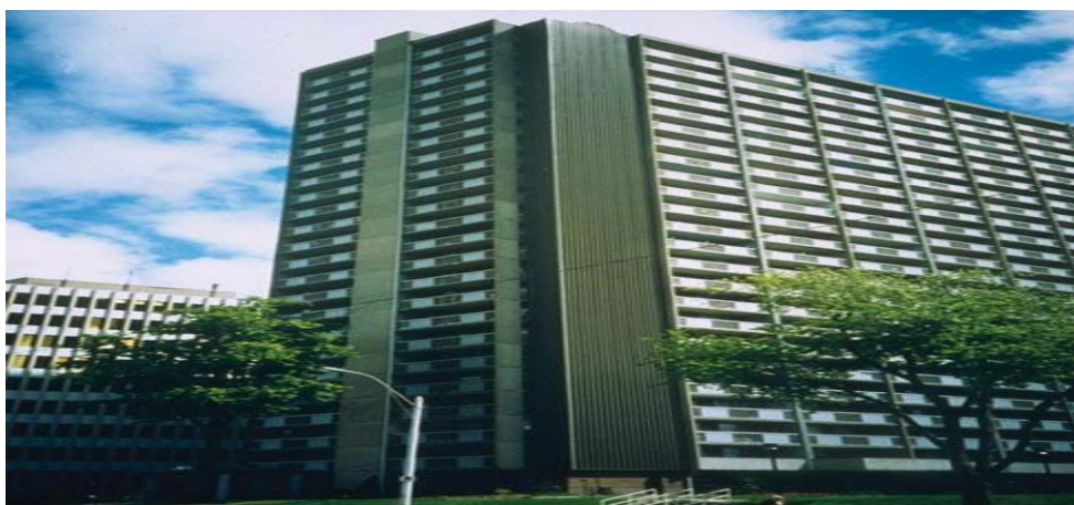
Figure 2.10: Multi-unit residential solar air heating project[8].
