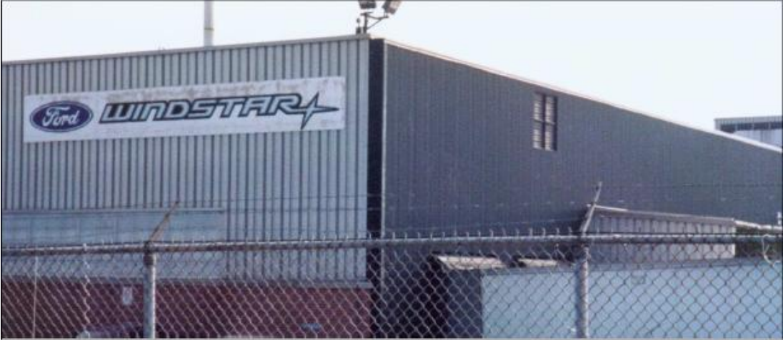
Figure 2.11: Oakville Assembly Plant [21].
