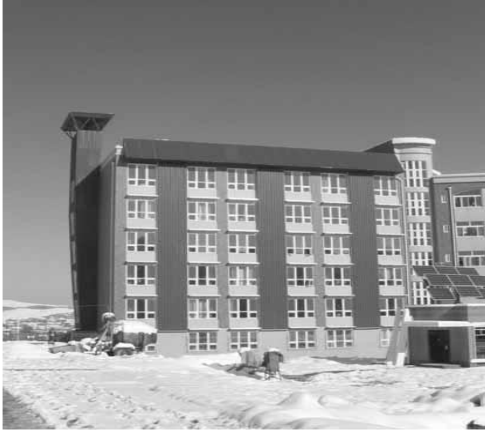
Figure 2.16: The appearance of the building [23].
