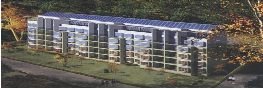
Figure 2.3: PV integration in a building [5].
