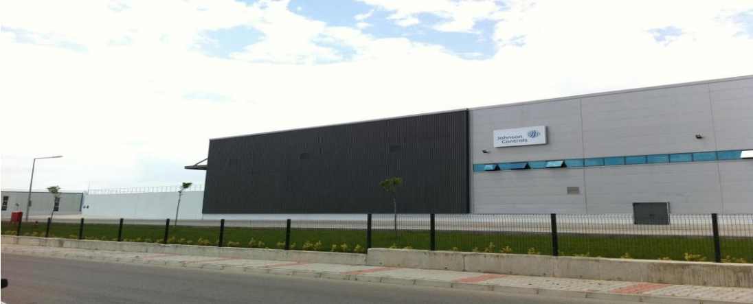
Figure 2.18: Unglazed transpired collector application in CRH group [24].
