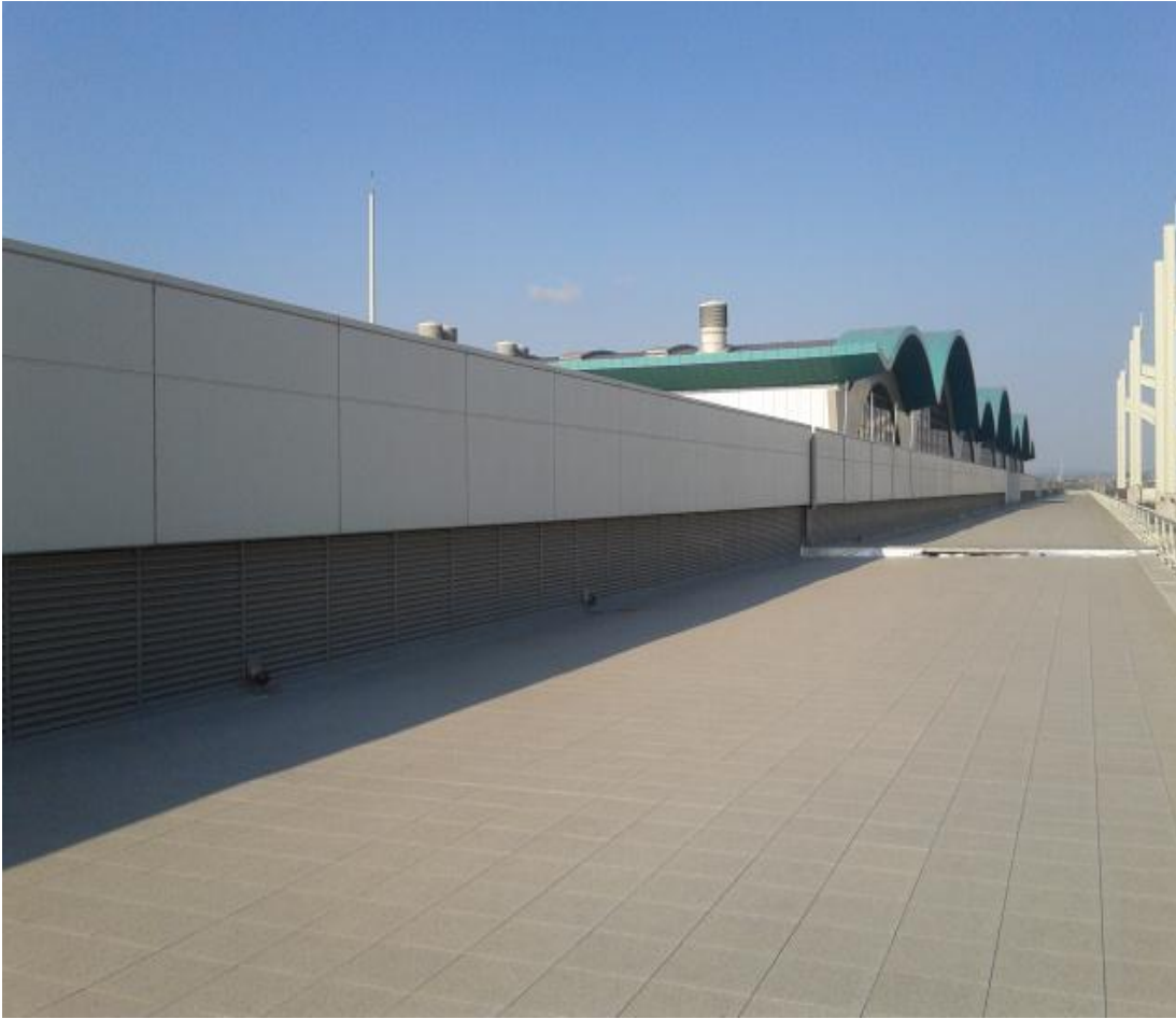
Figure 3.5: View of Mezzanine floor where Solarwall applied.
