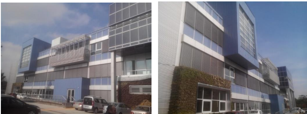
Figure 4.3 : Exterior photos of Ari 6 building.
