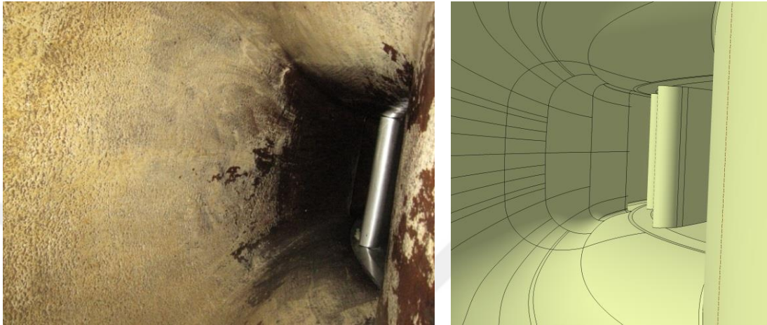
Figure 4.7 : Cutwater region of spiral case (left – reality, right – CAD model).
