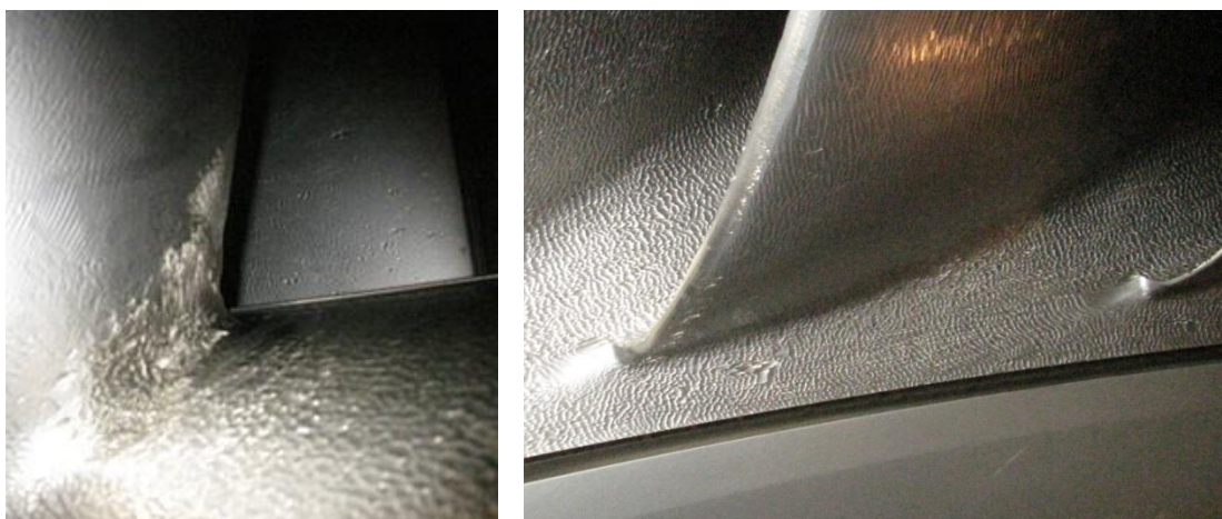
Figure 4.47 : Cavitation damages at the runner, leading edge (left), trailing edge (right).
