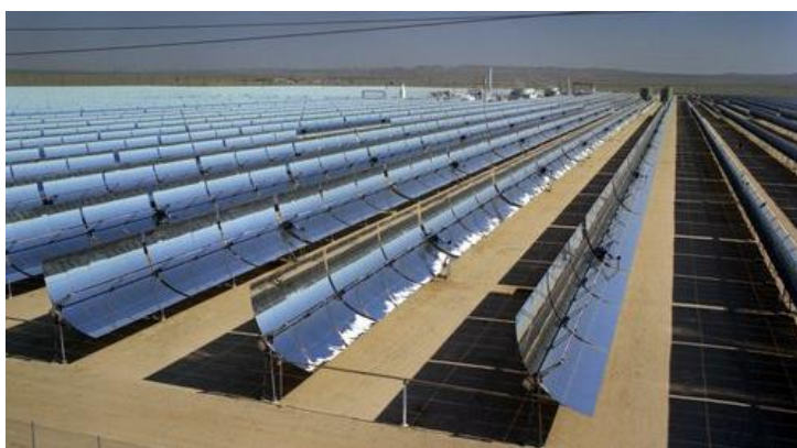
Figure 1.1 : Parabolic trough system (Khan et al., 2016).
