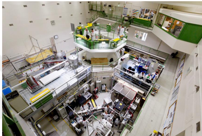
Figure 2.2 : Typical TRIGA Mark II Installation (Johannes Gutenberg University, Germany) [17].
