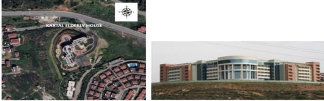
Figure 3.2: Views of building.
