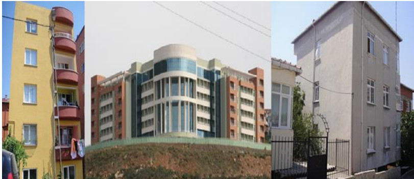
Figure 3.3 : External view of 3 buildings.
