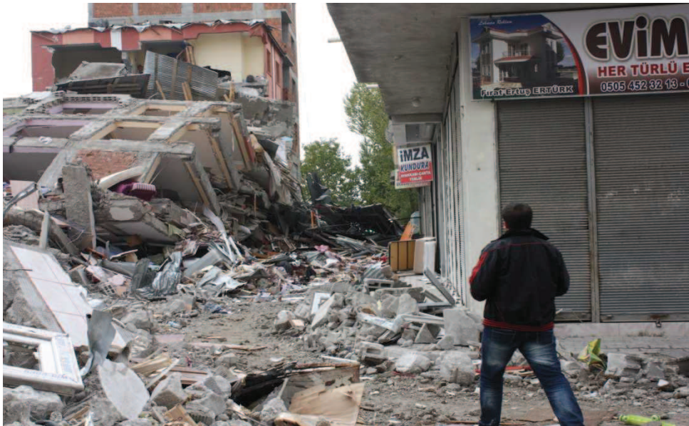
Fig 1. 23 October 2011 Earthquake in Van
