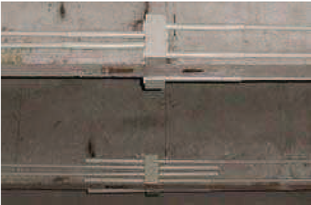
Fig.2.17. Typical Strengthening of External Post Tensioned Photo
