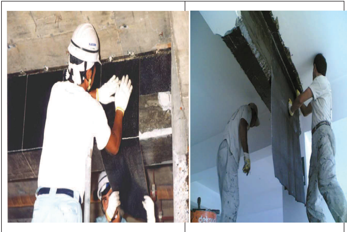
Fig.3.10. Application of FRP on reinforced concrete beams for seismic retrofitting
