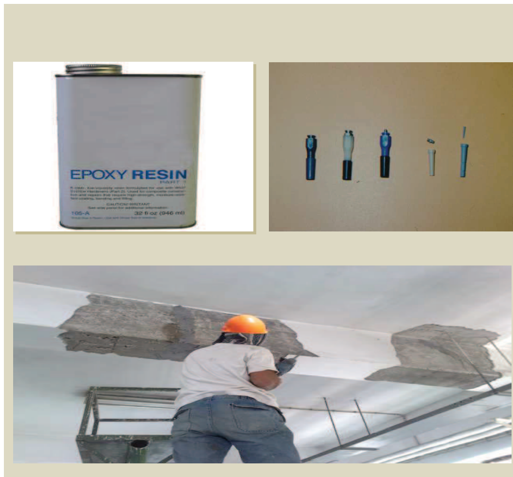
Fig.2.18. Epoxy resin ,injection port and application of epoxy resin
