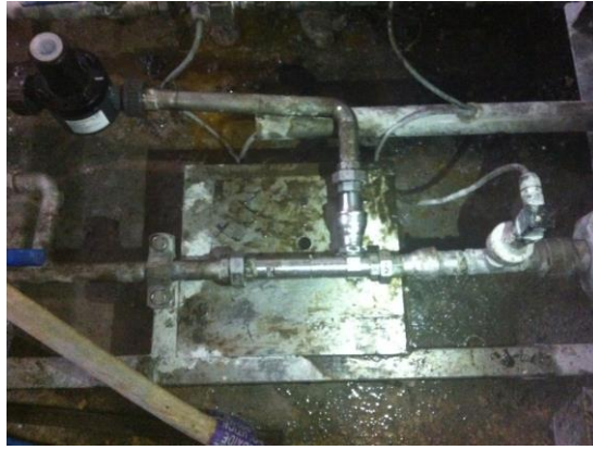
Figure 4.13 : Venturi injector with static mixing elements inside
