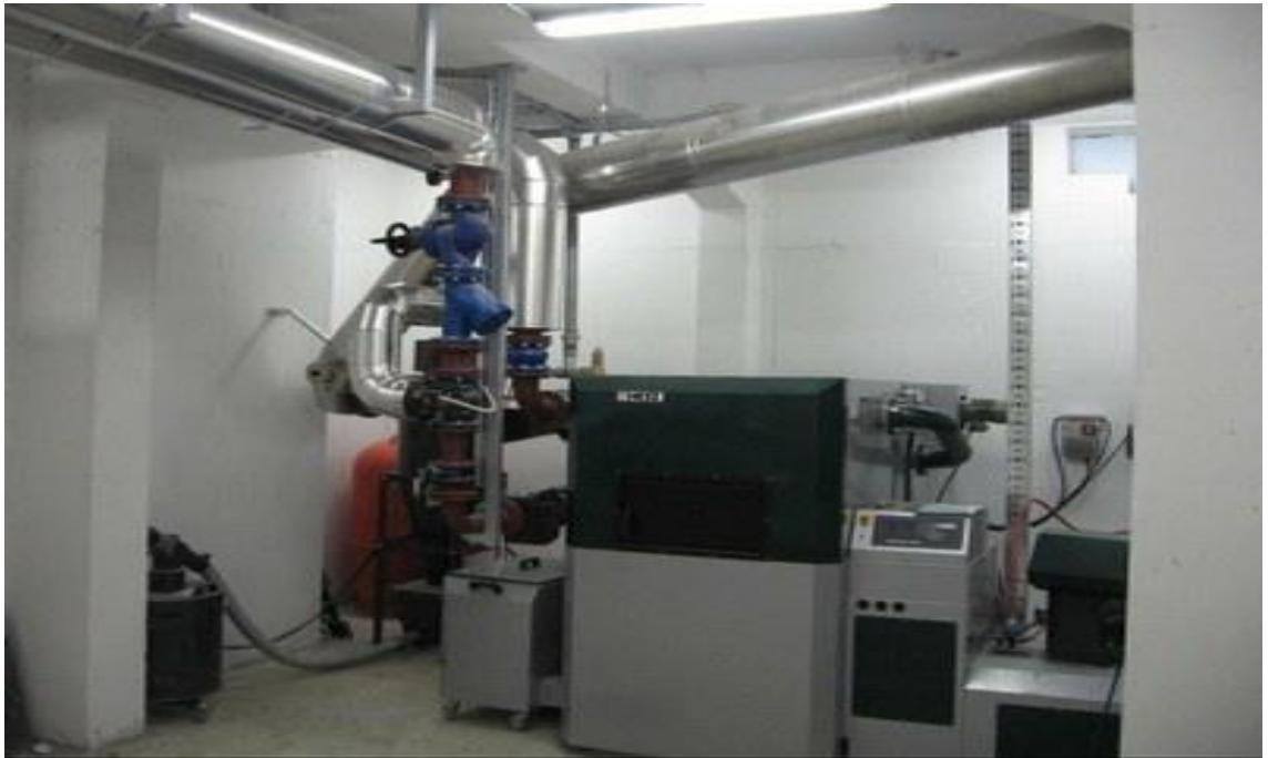
Şekil 2.101 Kazan, biyokütle kazan (www.alpstar-project.eu/cna-form/environment-friendly-and-energy-efficient-snovik-thermal-spa)
