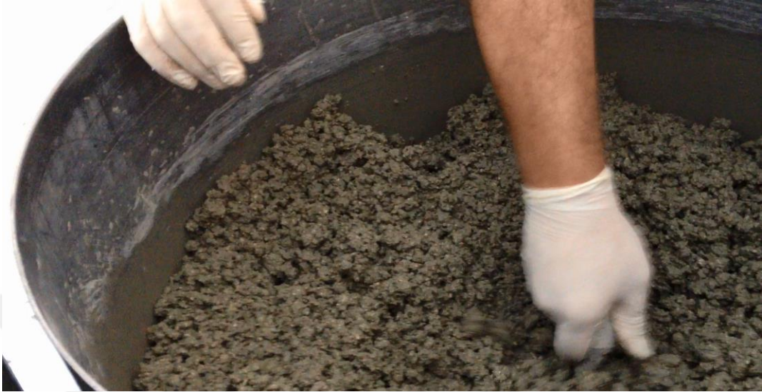
Figure B 1 Photographic view during concrete production
