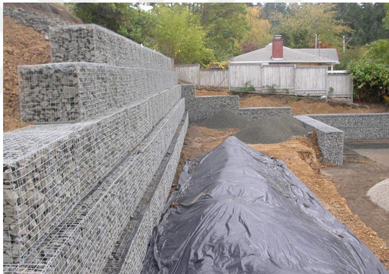
Figure 2.9 Gabion Facing ( http://www.kaengineers.com )
