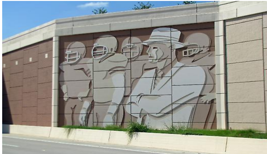
Figure 2.5 Facing element of MSE walls ( http://www.reinforcedearth.com )
