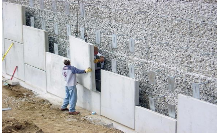
Figure 2.10 Post construction Facing ( http:// www.tensarcorp.com )
