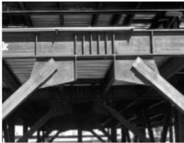
Figure 2.10 Eccentrically braced frame (Chimeh and Homami, 2012)
