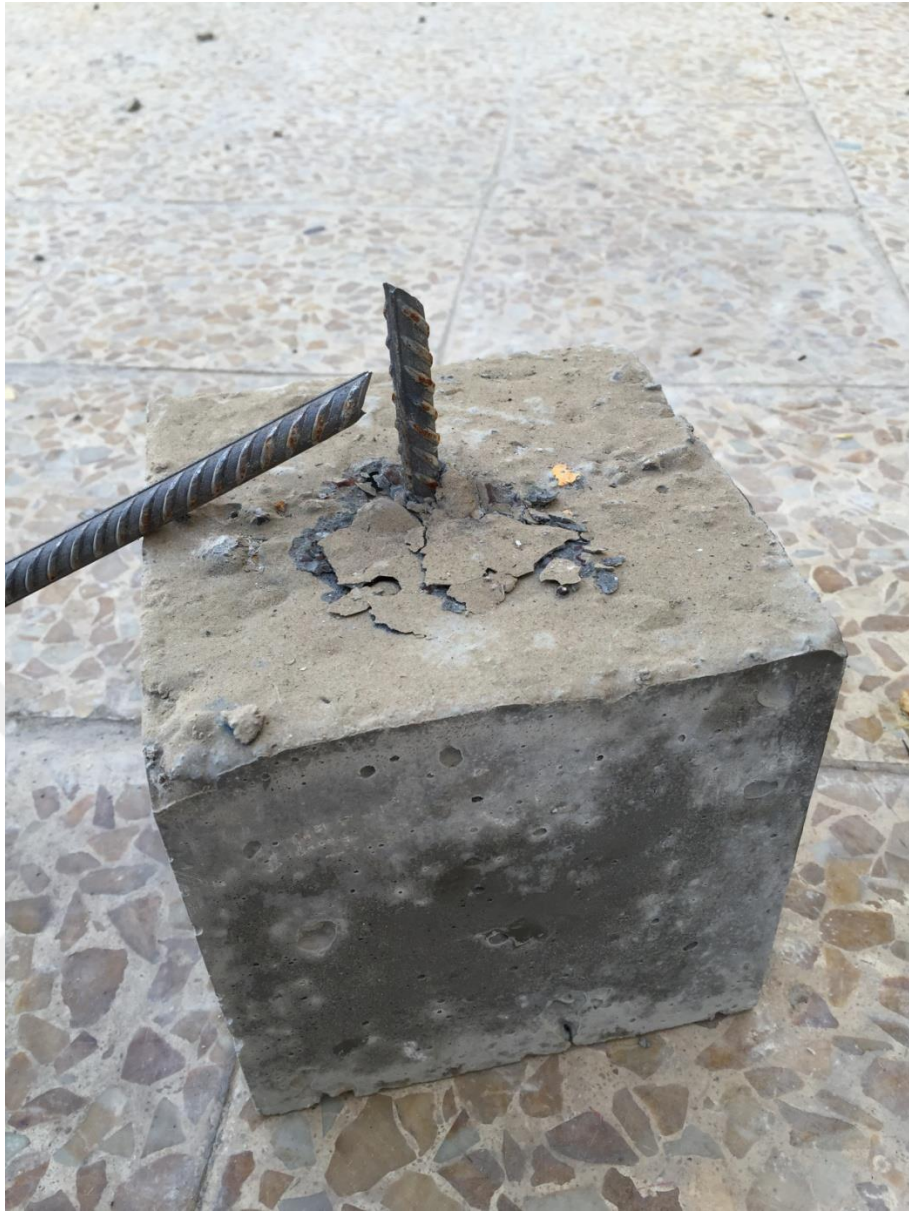
Fig (3.20) cut of the steel bar
