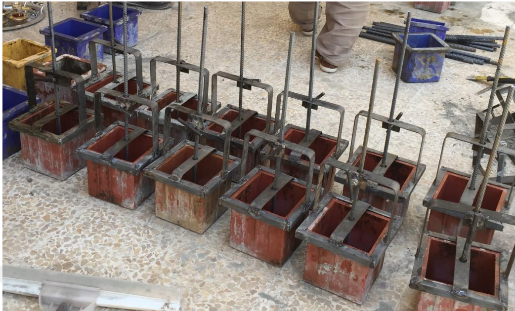
Fig (3.4) prepared the cube before casting Then with using an electric mixer as shown in Fig (3.5).
