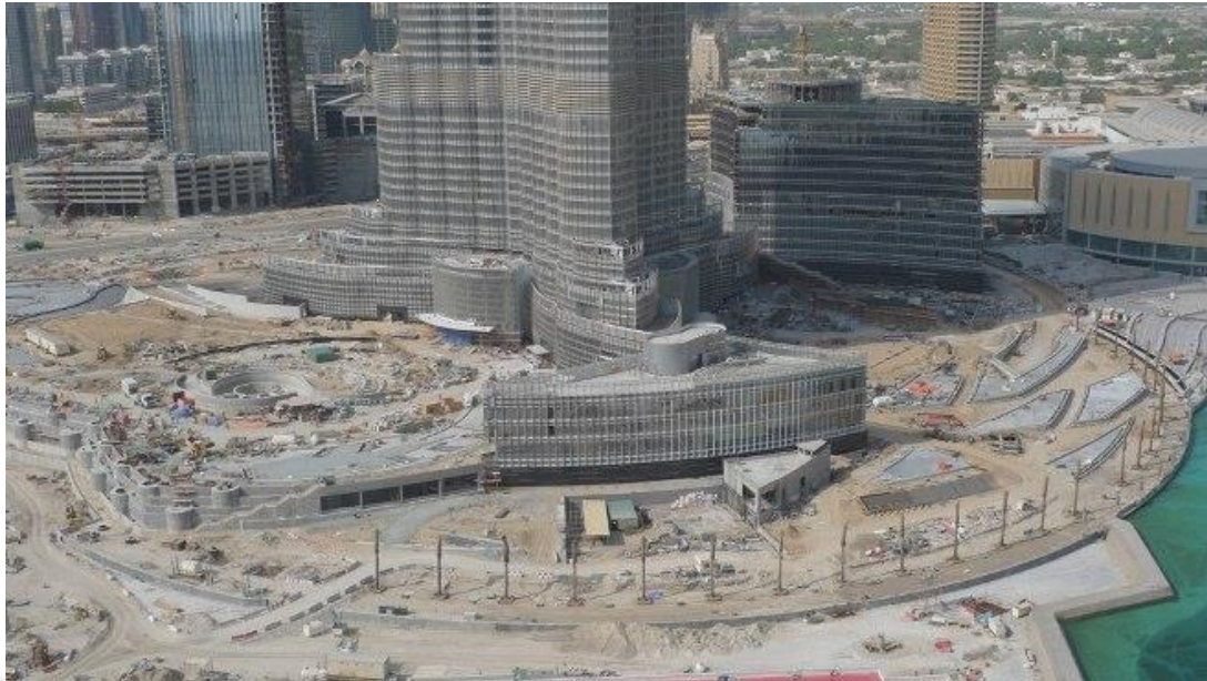
Fig. 2.12 Burj Dubai structure (Ruza, 2009)
