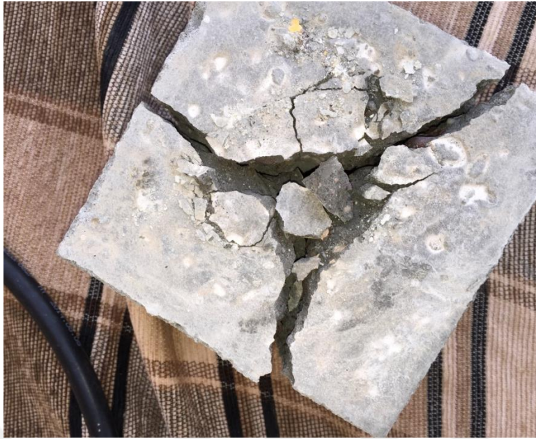
fig(3.18) failure concrete
