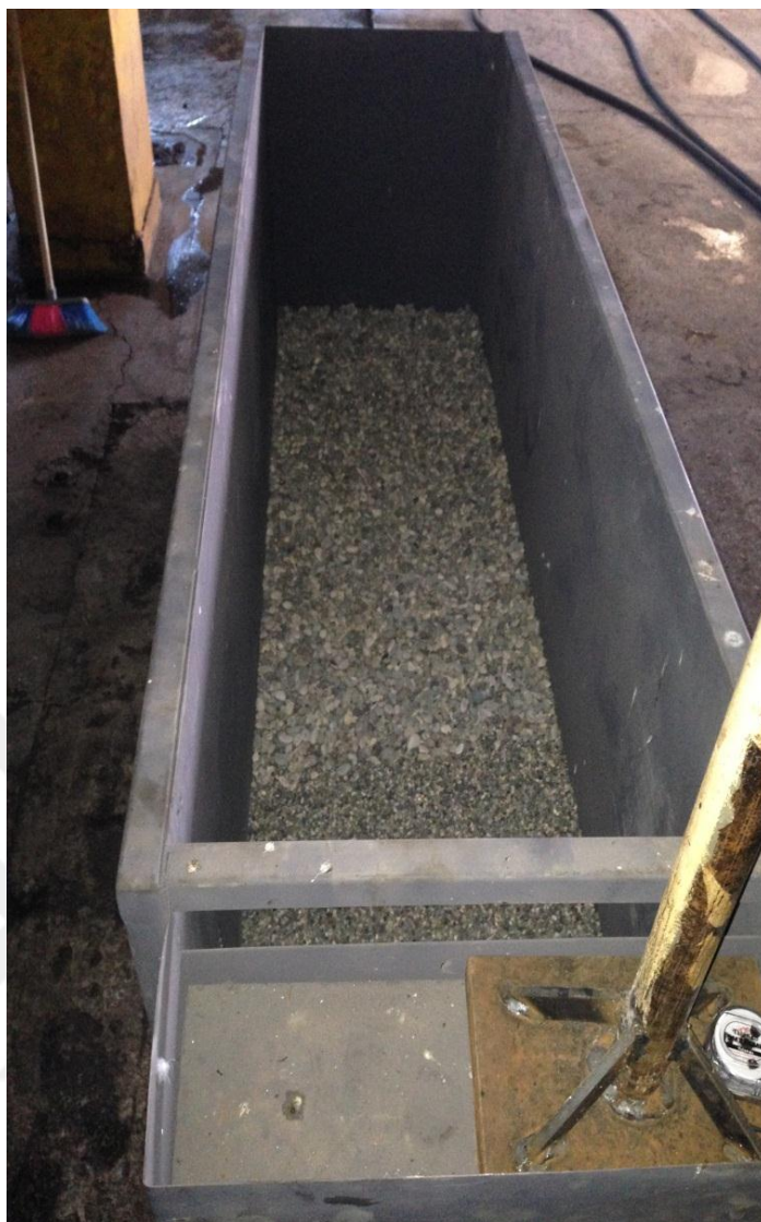
Figure 3.7 Gravel used for filtration
