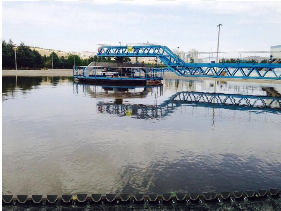
Figure 3.9 Last sedimentation tank of wastewater
