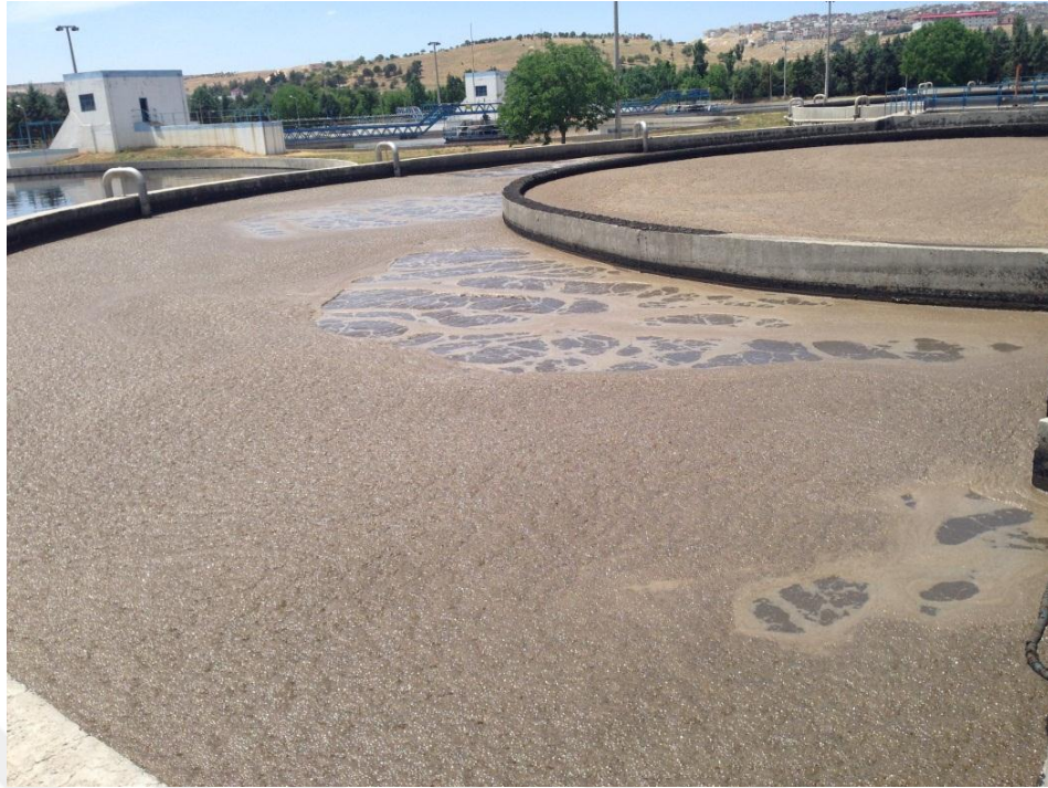
Figure 3.8 Wastewater treatment plant
