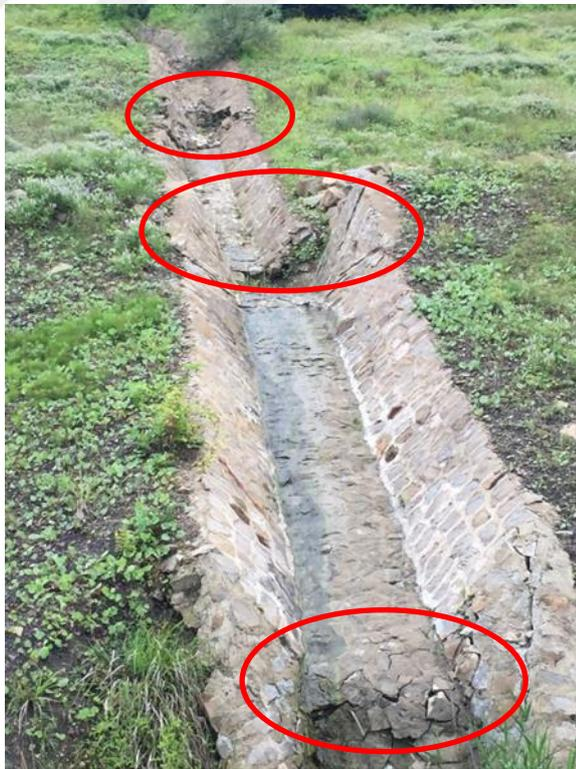
Figure 3.3 Damage at drainage lines due to landslide.
