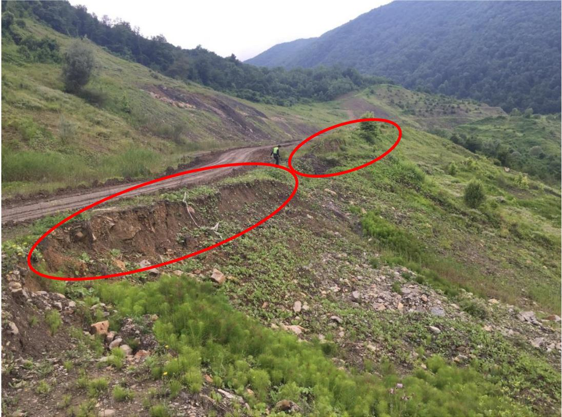
Figure 3.4 Movements at road level.
