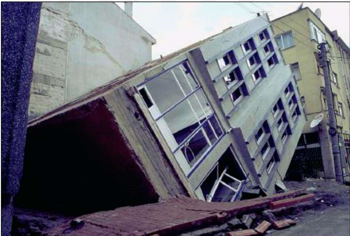
Figure 2.7. Soil's Loss of carrying capacity and building slanting (Ulusay, 2001).
