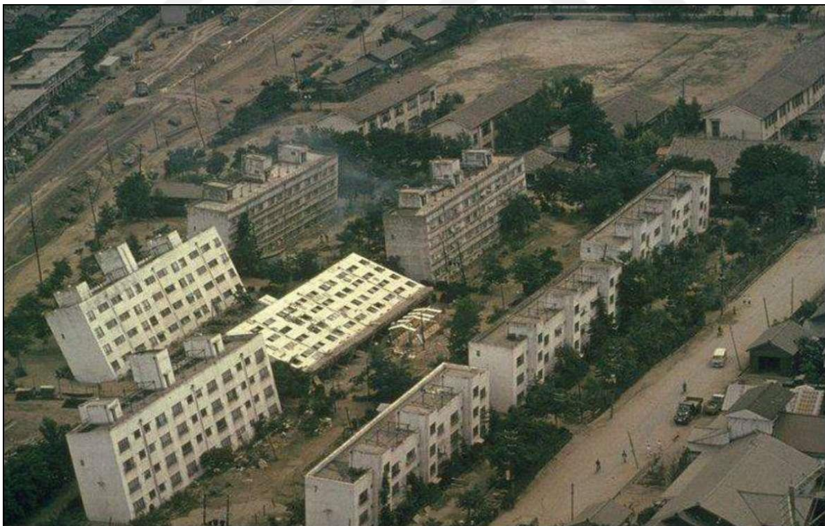
Figure 2.6. 1964 Buildings slanting and tumbling down by means of liquefaction in Niigata earthquake (Steinbrugge Collection, Earthquake Engineering Research Center, University of California, Berkeley) (Şen, 2004).
