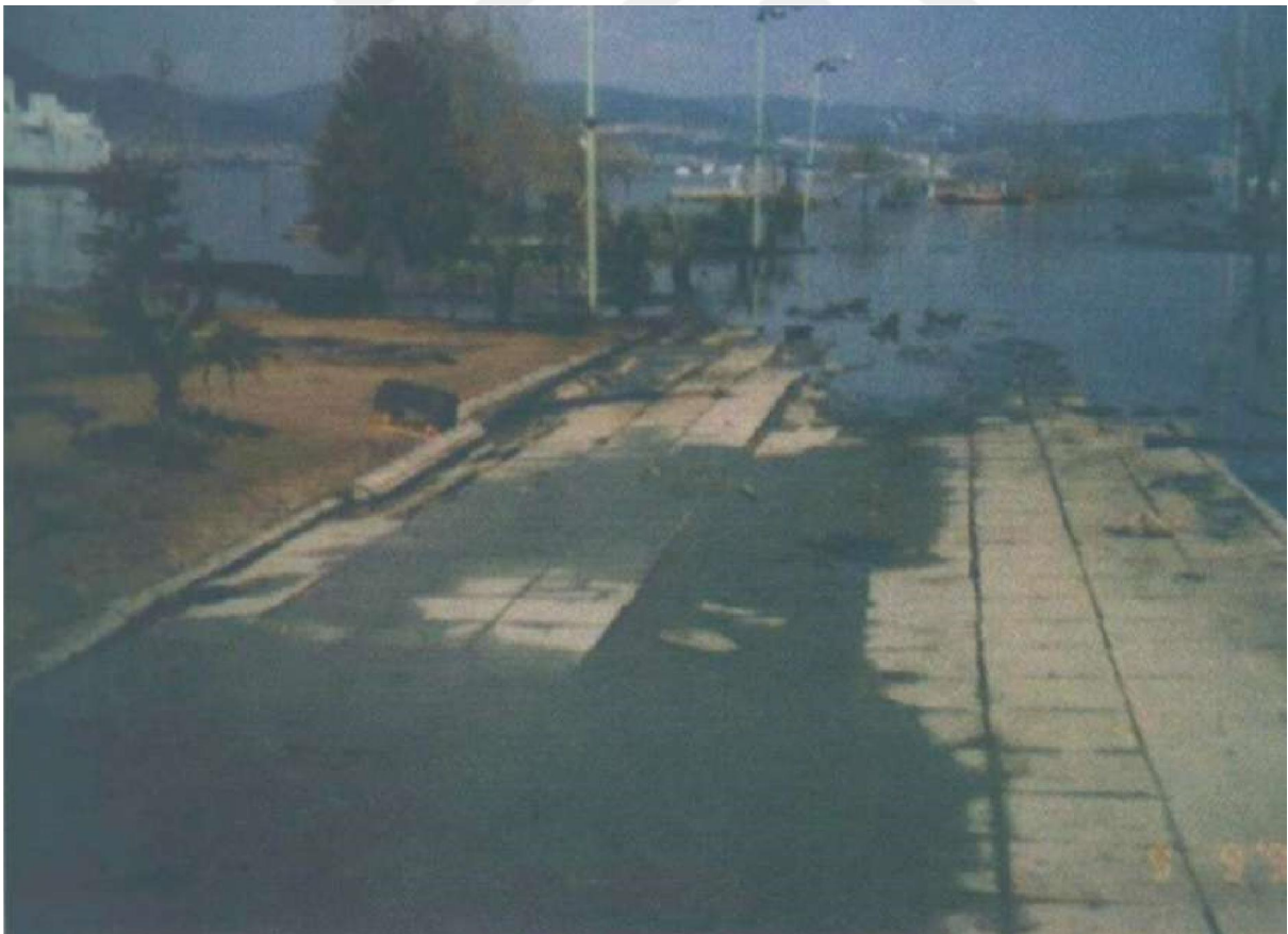
Figure 2.10. Development of Lateral Spreading (adapted from Obermeier, 1996).
