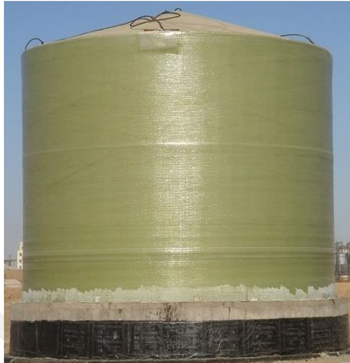
Figure 6. 22 Application of fibers on the cylindrical tank
