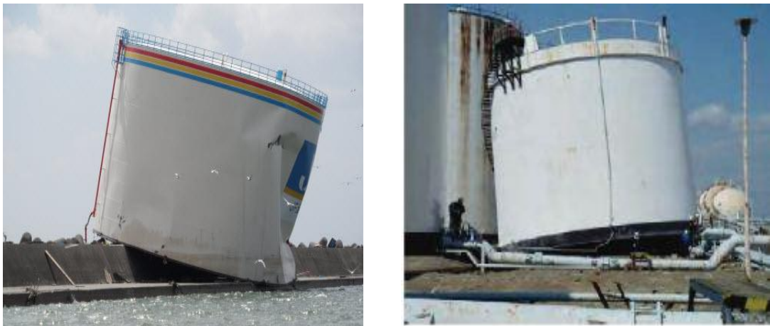
Figure 2. 5 Sliding and uplifting of tanks (Mohsen and Ali, 2015)
