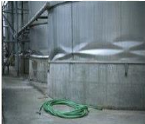
Figure 2.2 Diamond shape buckles (Mohsen and Ali, 2015)
