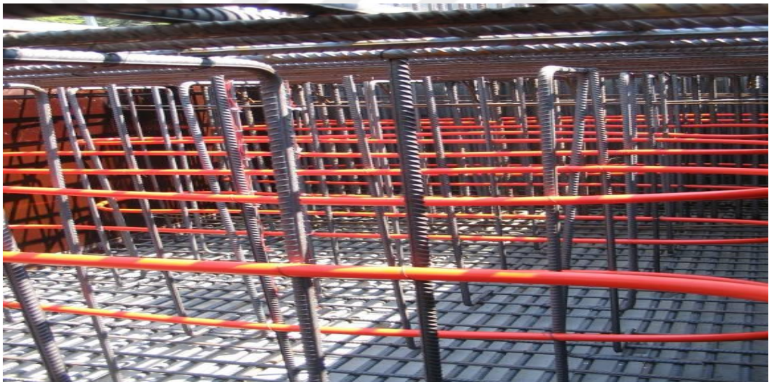
Figure 4.1. Post-Casting Cooling System Refrigeration (Cooling Pipes).
