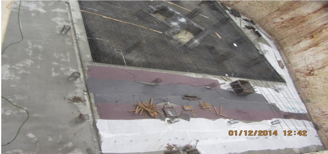
Figure 6.3. Concrete Casting Site
