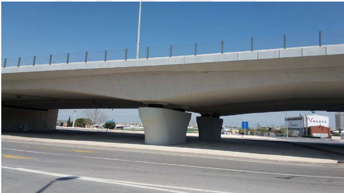
Figure 1.4 Denizli Market Hall Junction Bridge Middle Support
