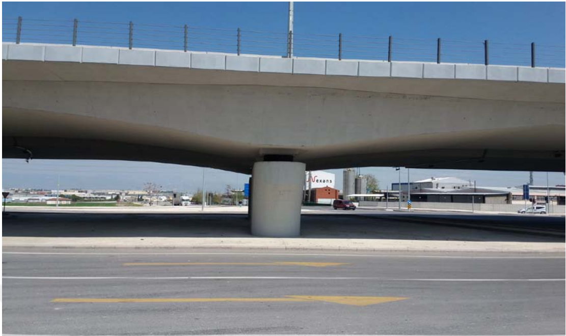
Figure 1.3 Denizli Hal Junction Bridge Middle Foot
