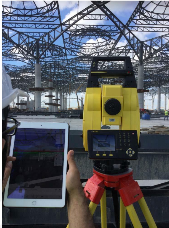
Figure 22: BIM Site controlling & installation with BIM360 layout application
