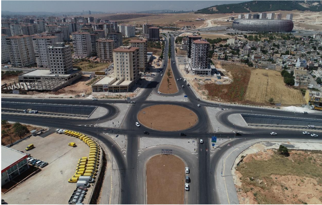
Figure 3.6: Beykent Bridge Crossing-2, Gaziantep, Turkey
