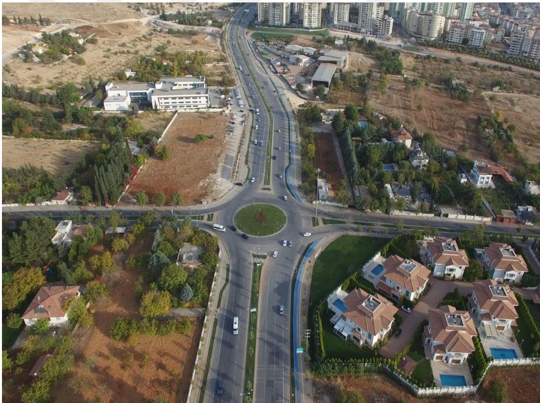
Figure 3.4: Nijmegen Roundabout, Gaziantep, Turkey
