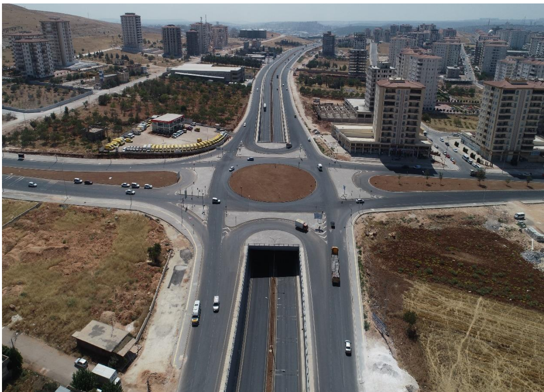
Figure 3.5: Beykent Bridge Crossing-1, Gaziantep, Turkey
