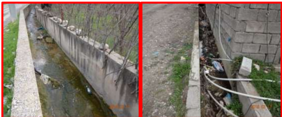
Figure 4.10 Rubbish convey to the irrigation canal and to the houses water use
