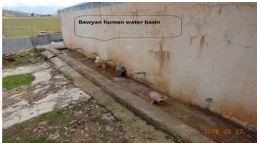
Figure 4.7 Household concrete water basins, Bawyan village
