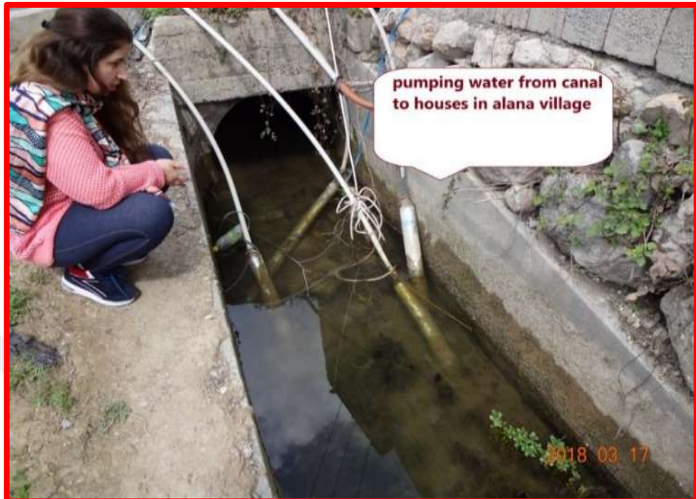
Figure 4.11 Pumping water and supply from the water canal to the houses use
