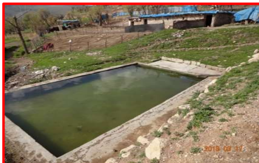
Figure 4.12 Concrete water basins for domestic water use
