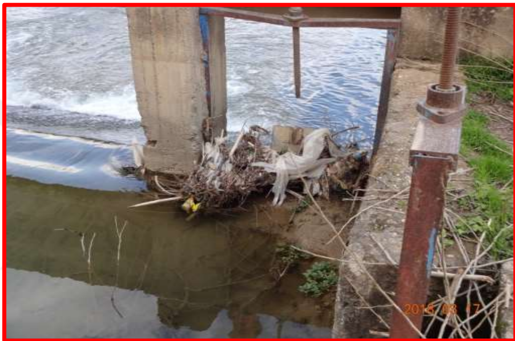
Figure 4.9 Alana irrigation project, weir structure
