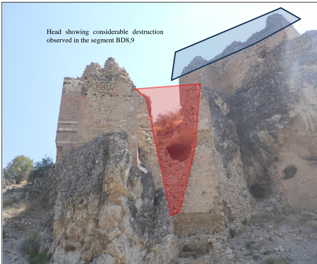
Figure 14. Irregular Demolition in Western Front, BD-8, 9
