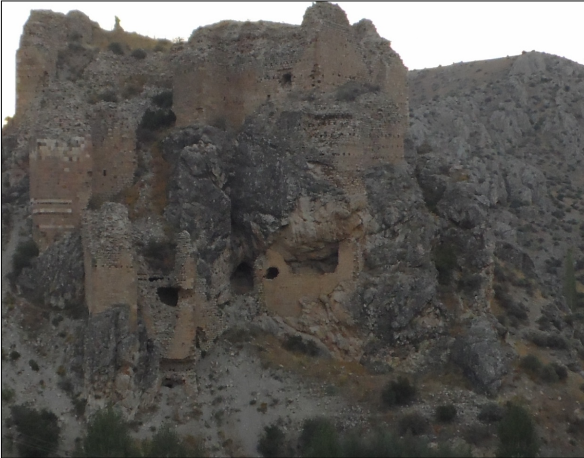
Figure 15. Non-Plane Demolition of Long Span Wall Segment in the Western Front and BD-6 Wall
