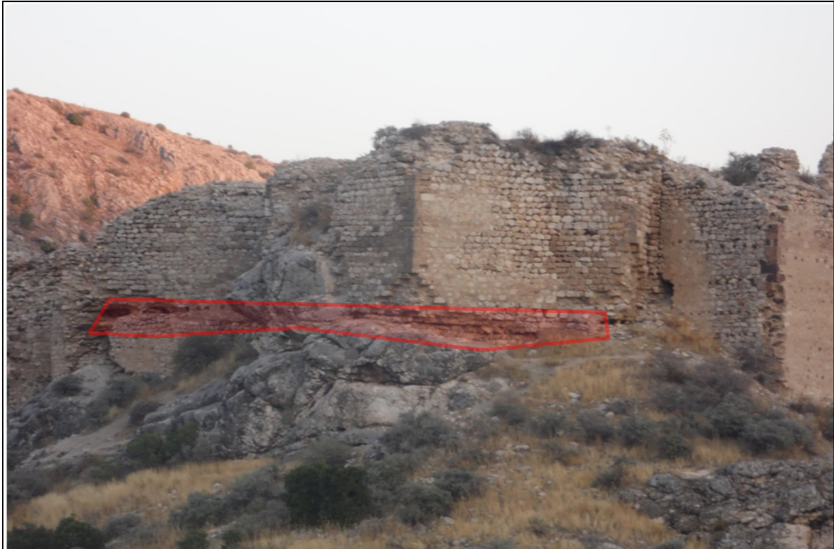
Figure 9. The Downward Trench Level External Wall Loss from the GD-8 Wall to the DD-16 (Eastern Corner Wall) on the Southern Exterior Wall
