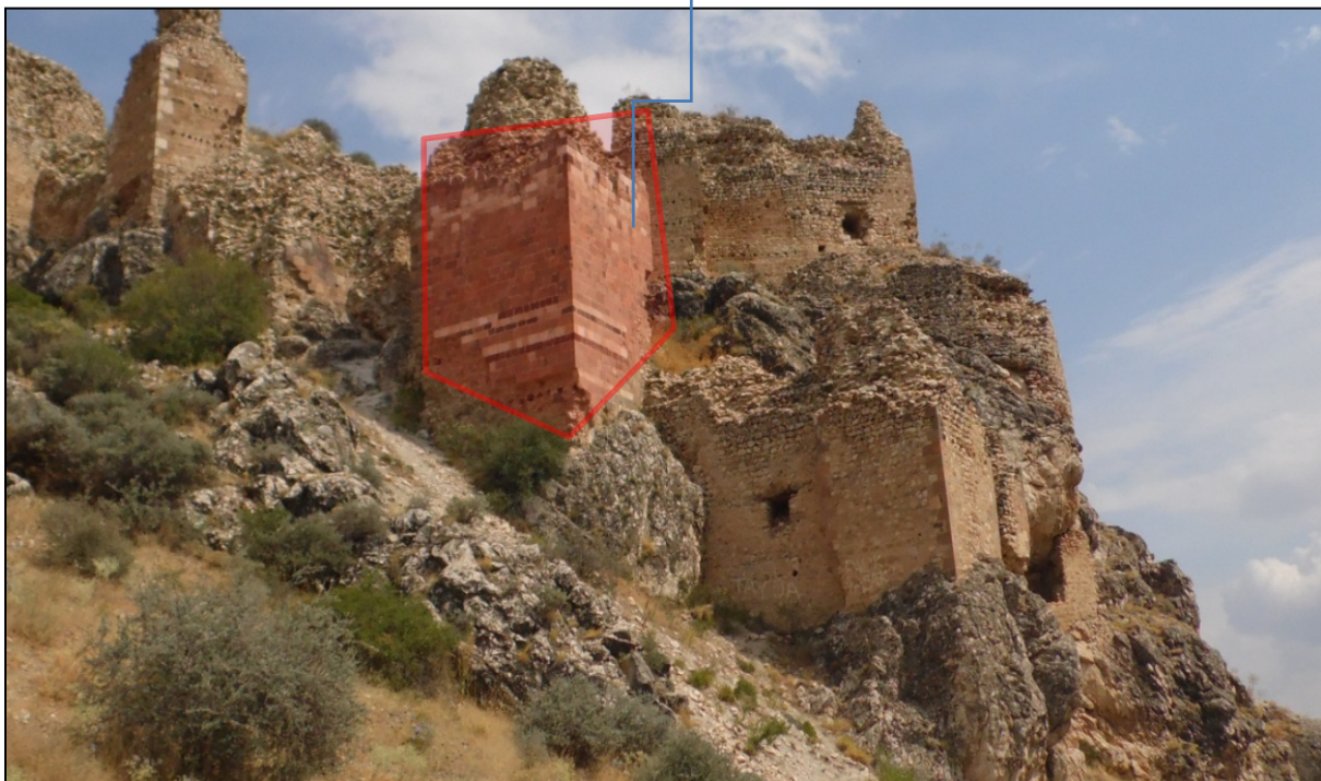
Figure 11. North Wall Exterior, West Slope Segment View
