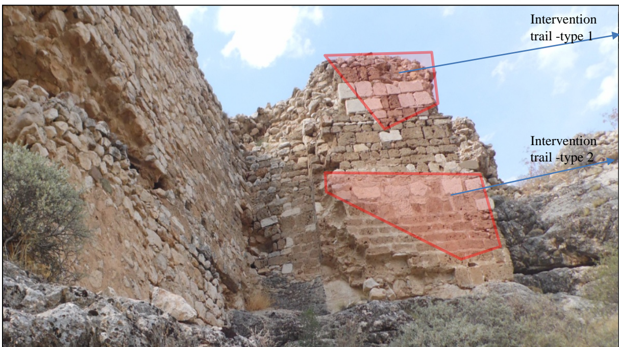
Figure 8. Sampling of Periodic Weave Differences or Repairs Detected on Southern Exterior Walls
