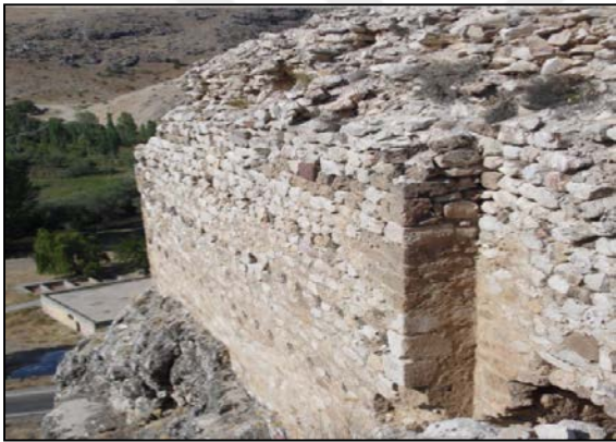
Photo 2. Hurman Castle a) Exterior wall structure in the outer wall structure, wooden vertical chain systems and internal rubble filling upper elevations of the observation. b) In the interior vault stone lattice, deterioration is observed with the eye eye condition. Travertine type stone material is a common type of decay.
