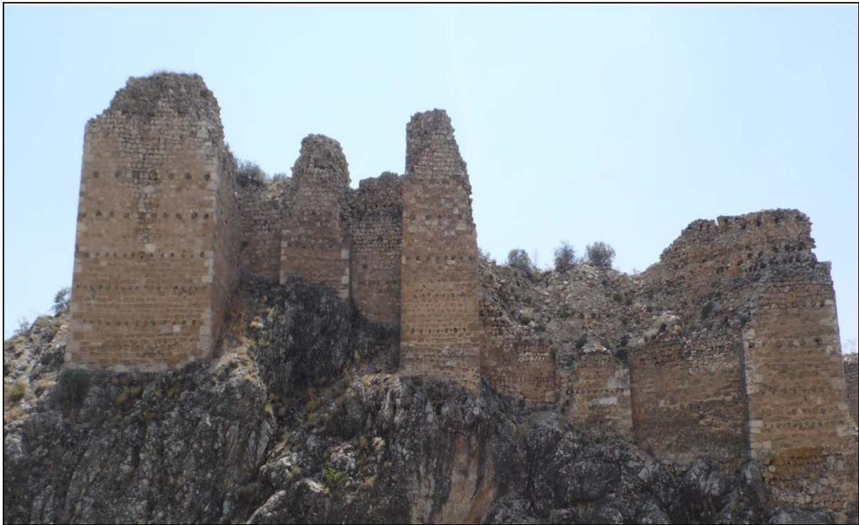
Photo 6. North Wall Exterior View
