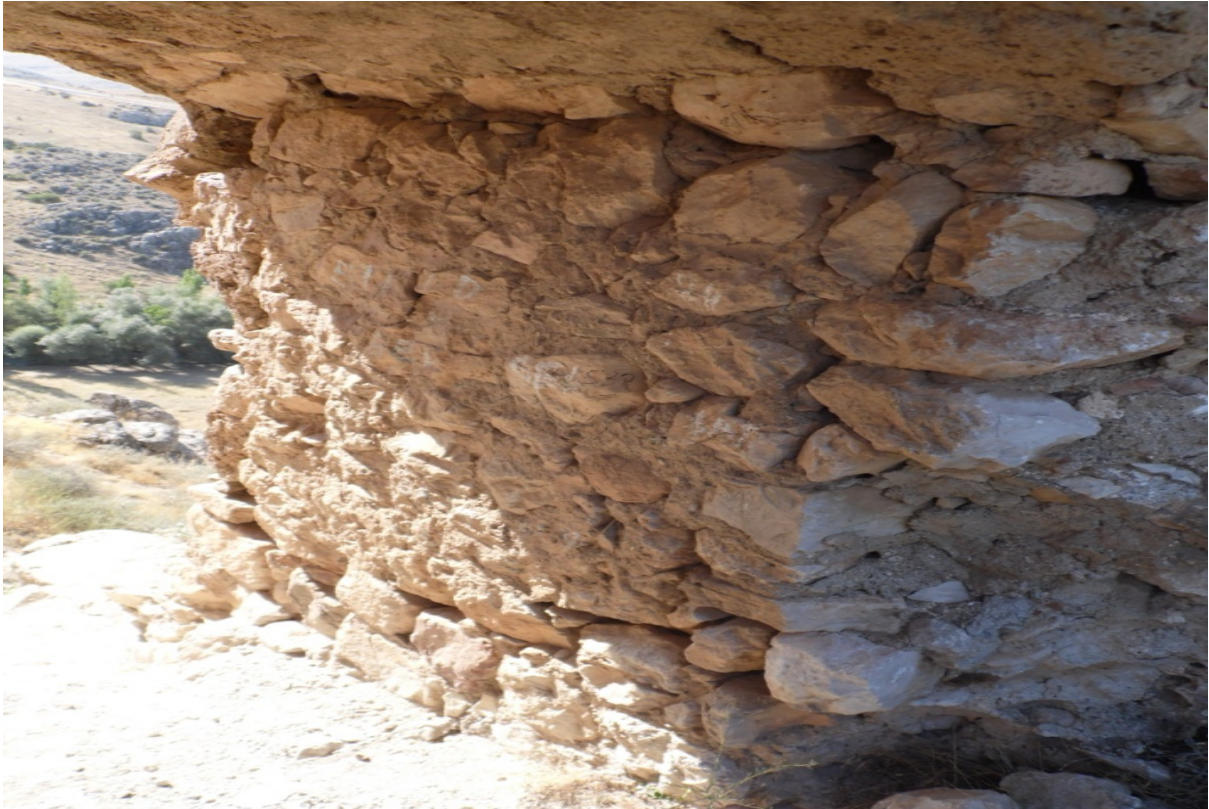
Photo 12 . Cross Section AA (South Front) Entrance
