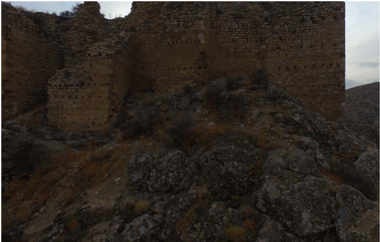
Photo 68 . Wall of DD 1-3-5-7-8-9-11-12
