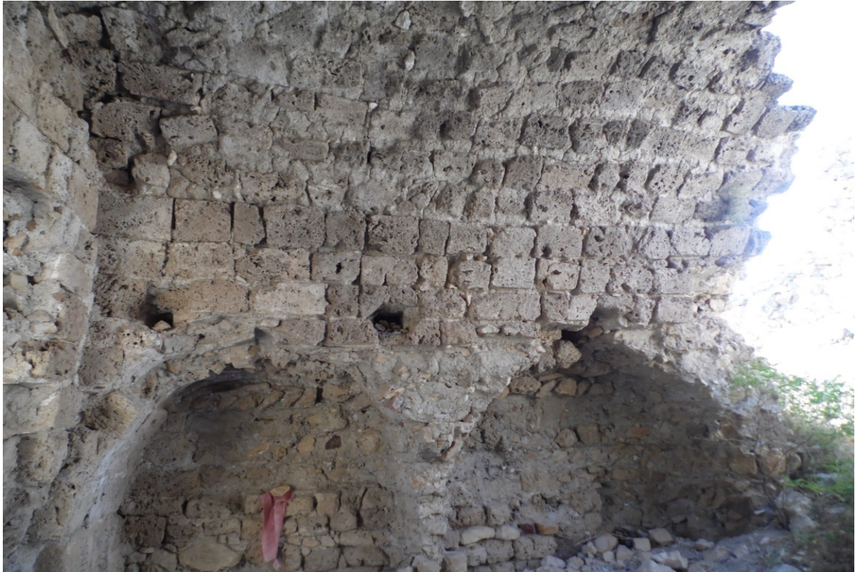
Photo 18 . Tower South Wall (Section 5-5)
