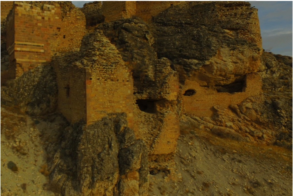
Photo 43 . A North View of the Lower Western Wall
