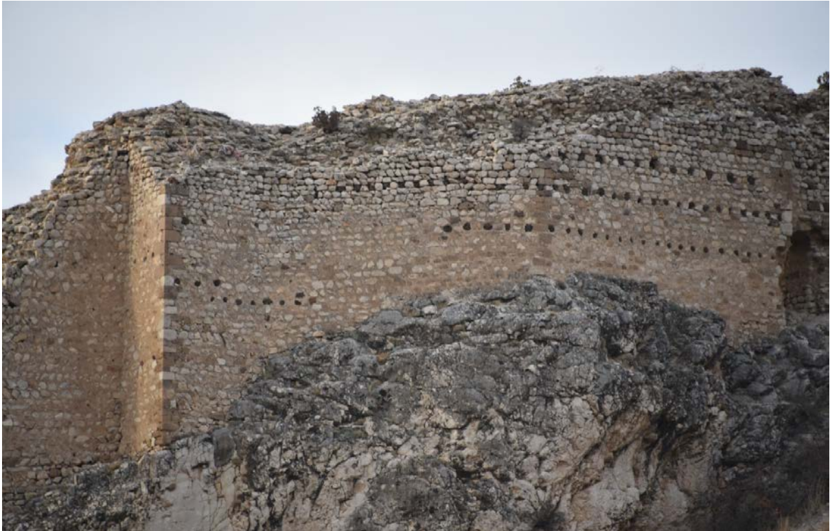
Photo 88 . Wall of GD 15-16-17-18-19
