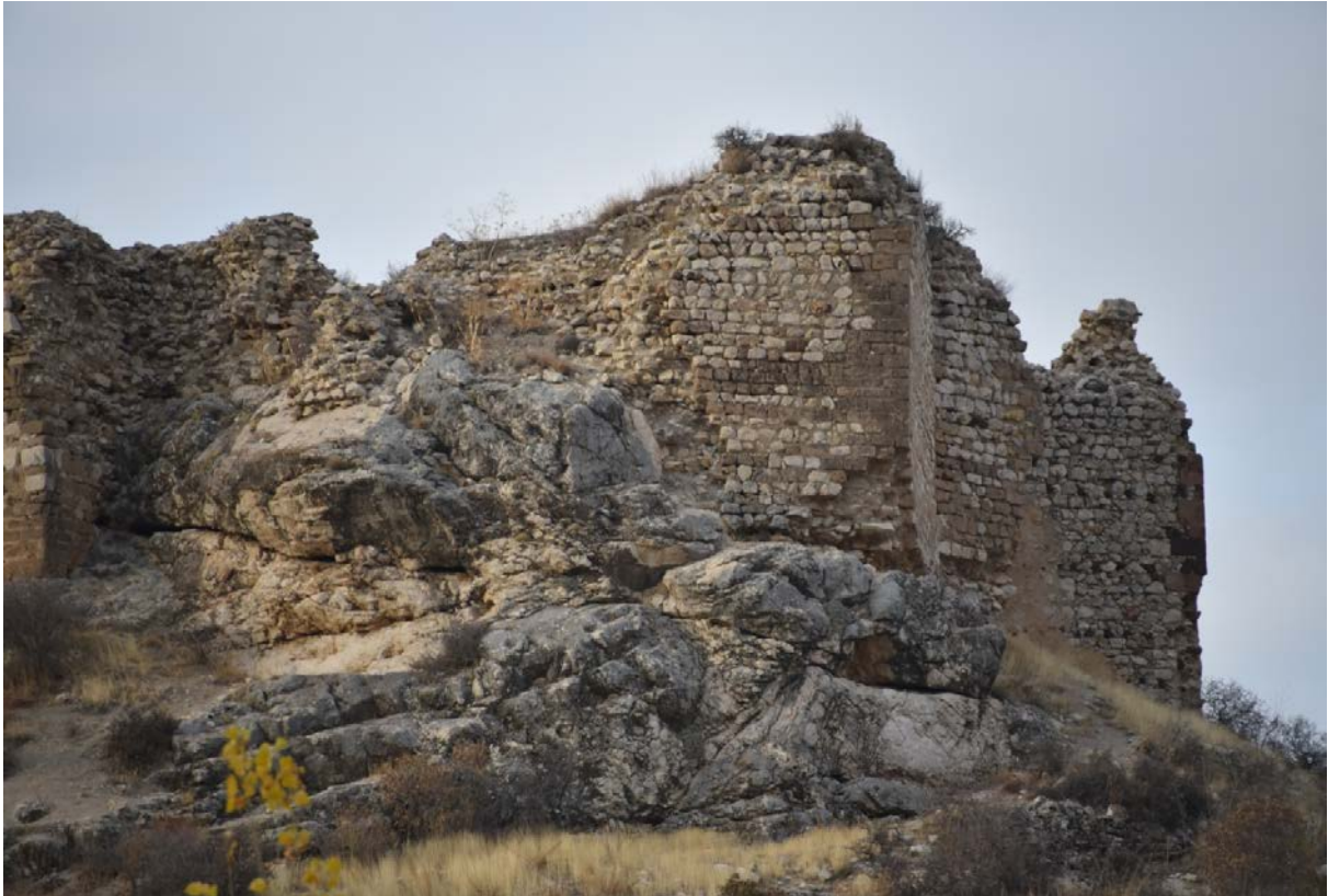
Photo 80 . Wall of GD 1-2-3
