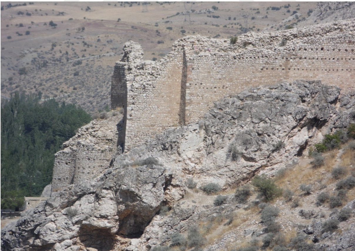
Photo 89 . Wall of GD 15-16-17-19
