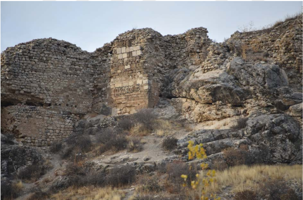
Photo 81 . Wall of GD 3-4-5-7-8
