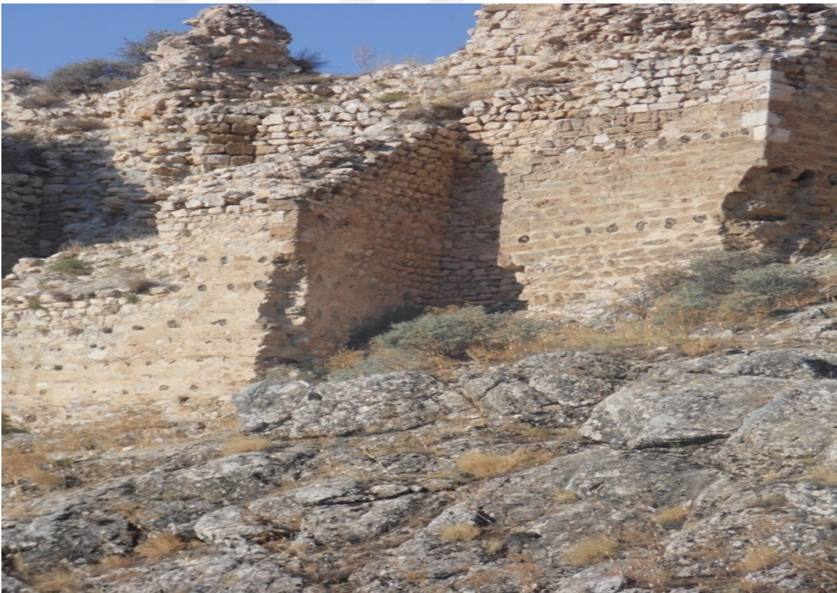
Photo 70 . Wall of DD 7-8-9
