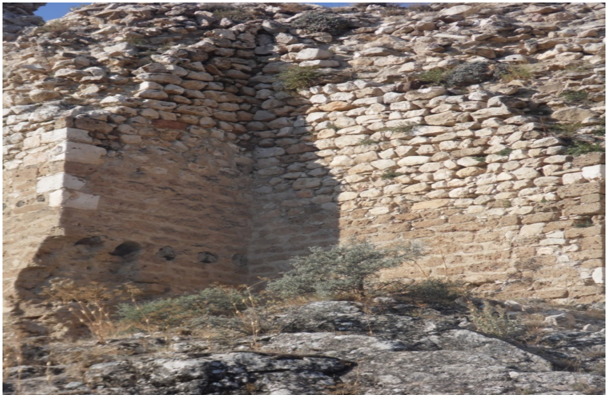
Photo 66 . Wall of DD 3-4
