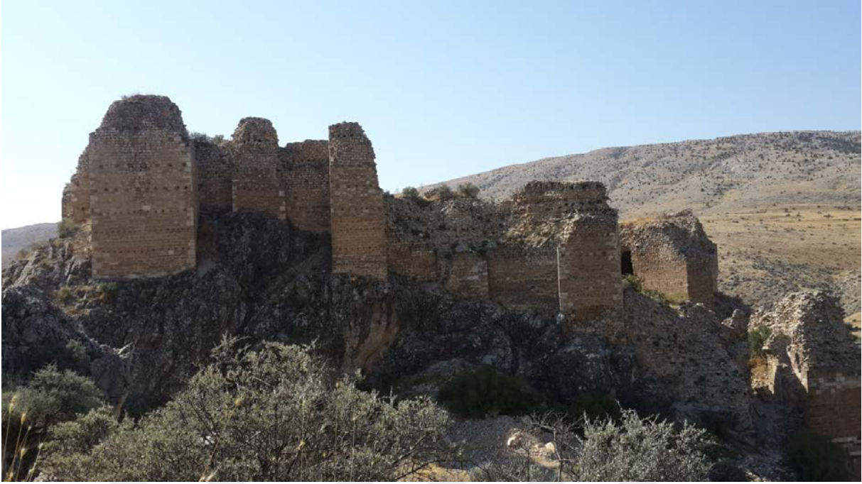
Photo 93 . North Side East Section
