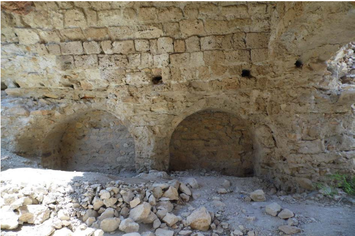
Photo 23 . Tower North Wall (Section 6-6)
