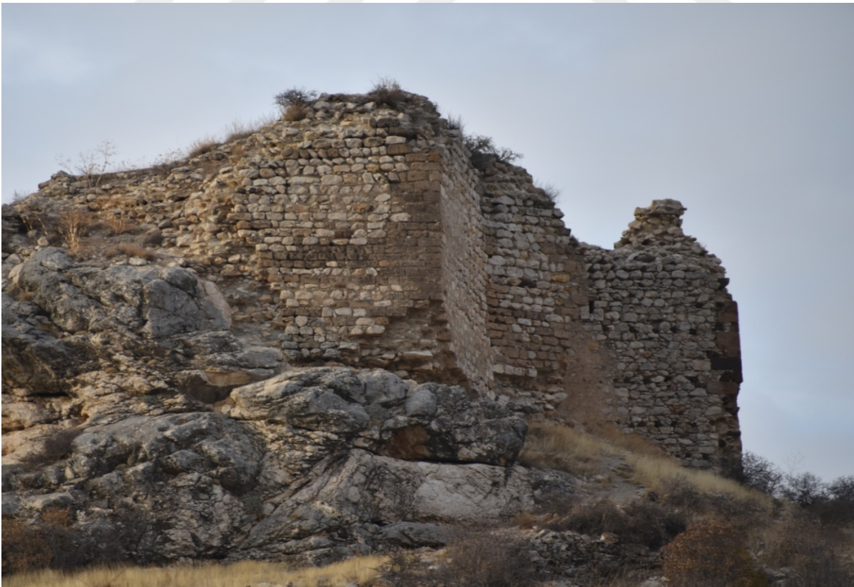
Photo 74 . Wall of DD 14-16
