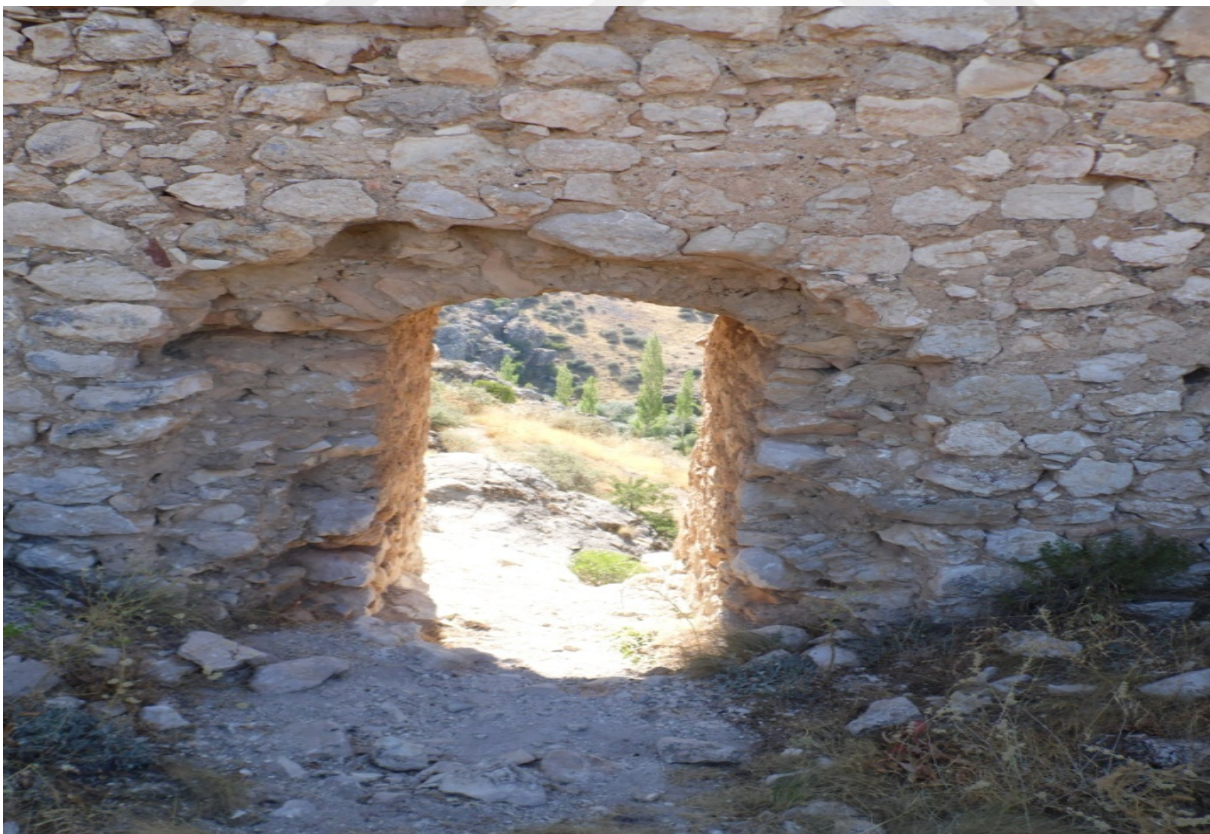
Photo 11 . Cross Section AA (South Front) Entrance
