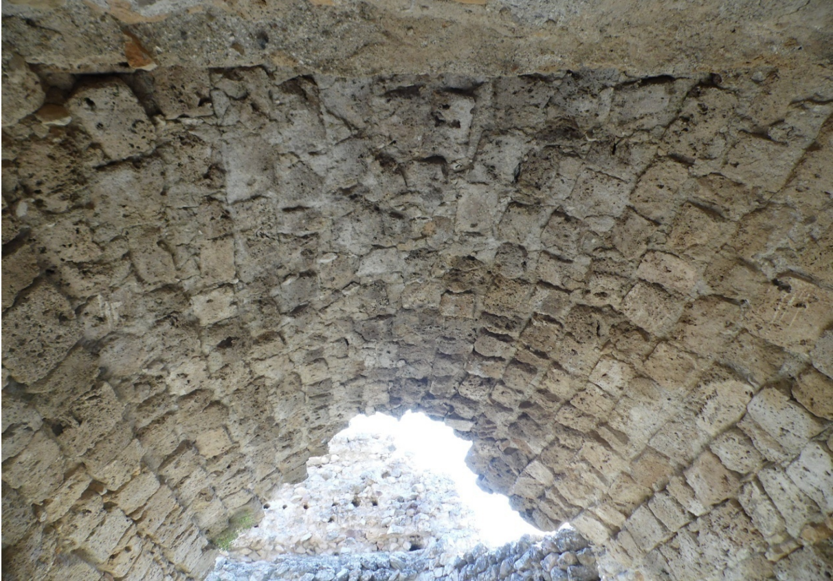
Photo 20 . Tower Western Wall (Section 8-8) and Stone Vault
