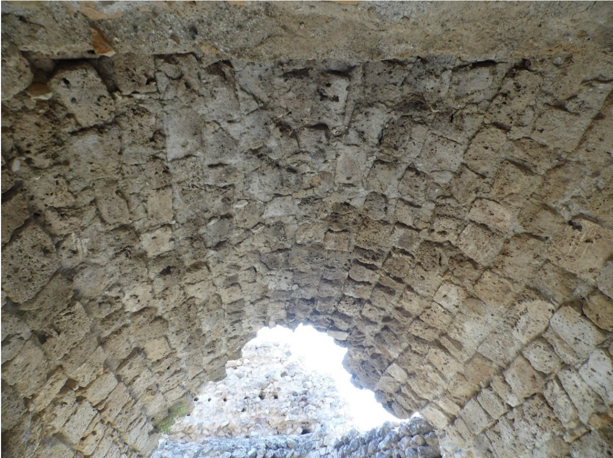
Photo 26 . Tower Stone Vault (West View)
