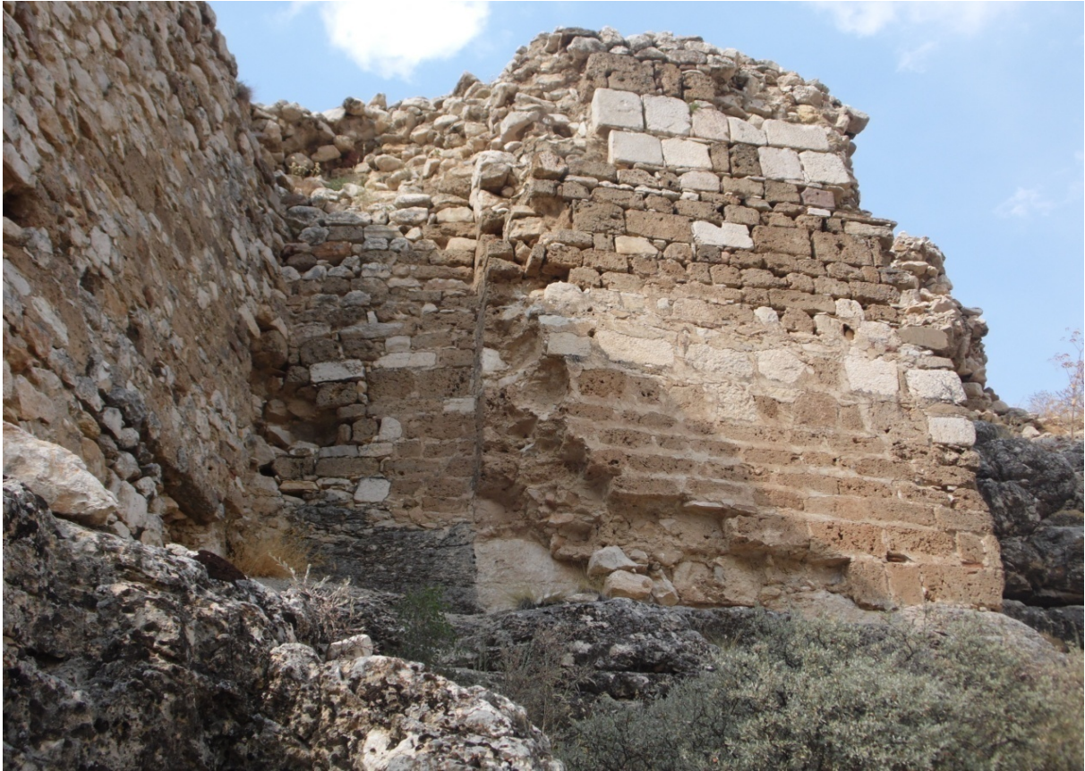
Photo 82 . Wall of GD 5-7
