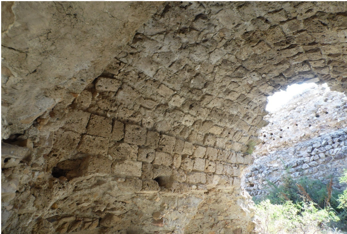
Photo 19 . Tower South Wall (Section 5-5) and Stone Vault
