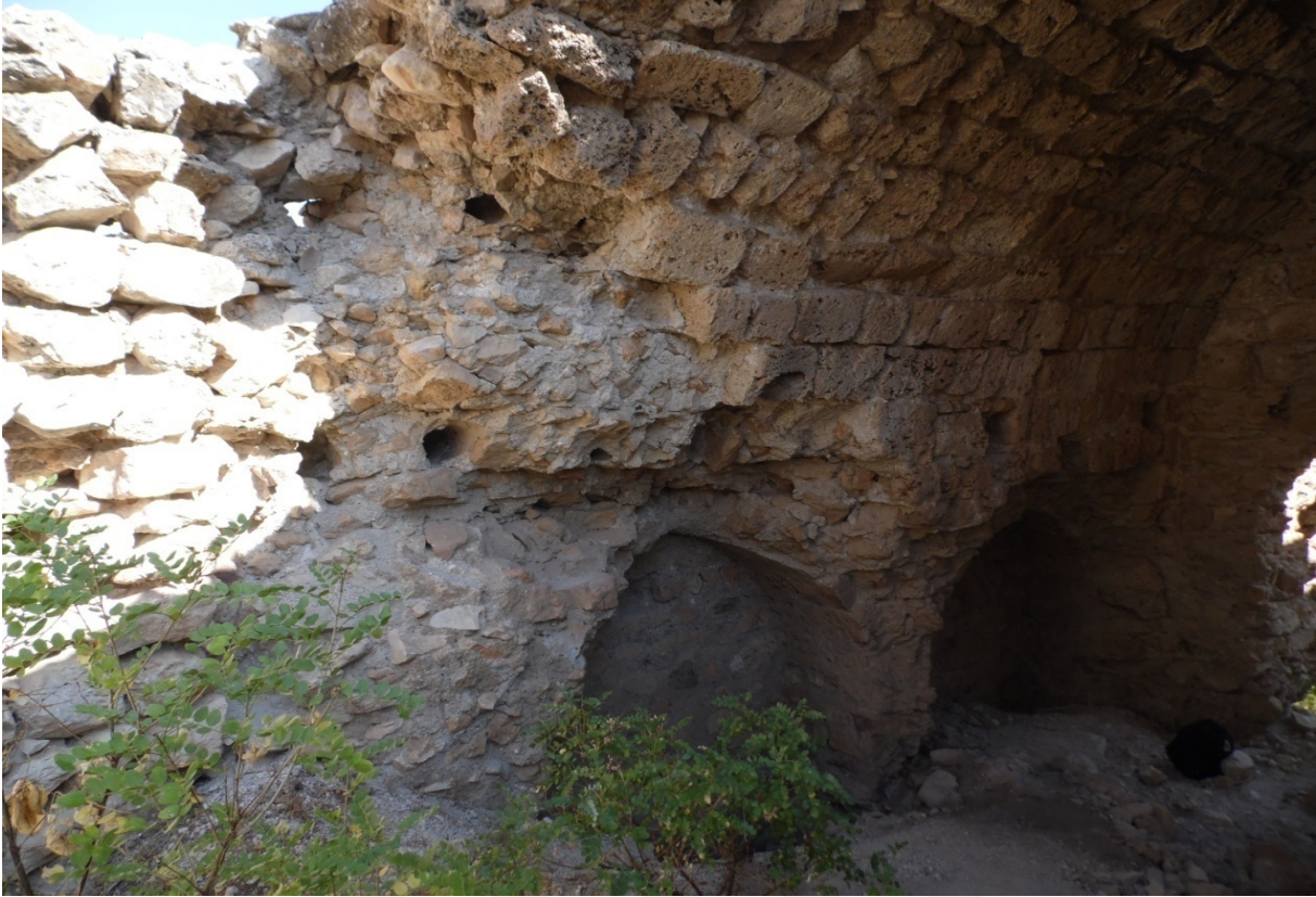
Photo 22 . Tower North Wall (Section 6-6)
