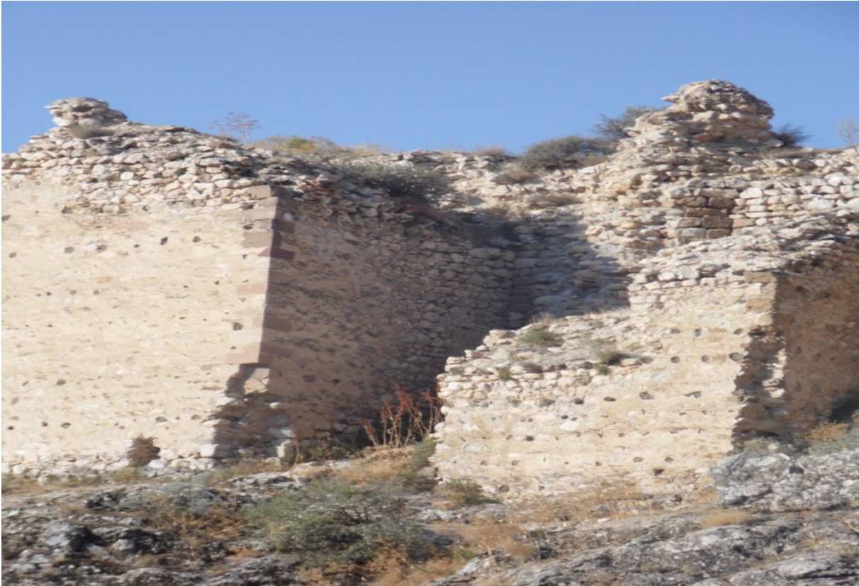
Photo 71 . Wall of DD 9-11-12-13
