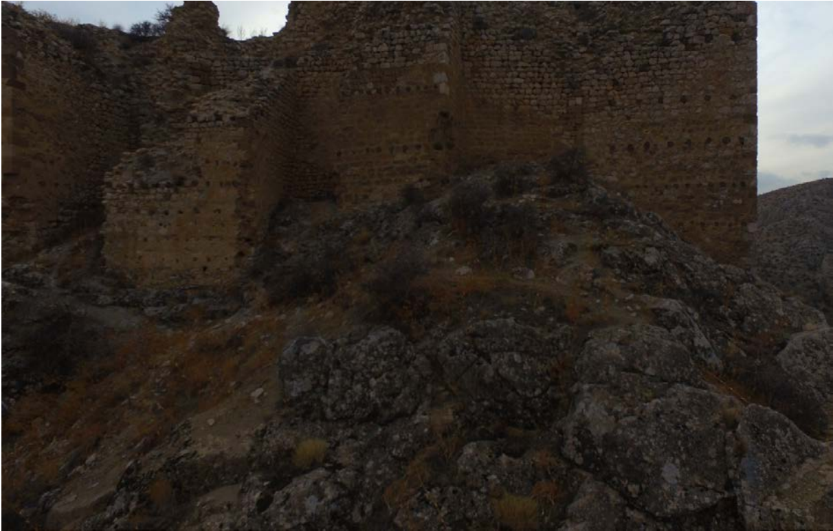
Photo 69 . Wall of DD 1-3-5-7-8-9-11-12-13
