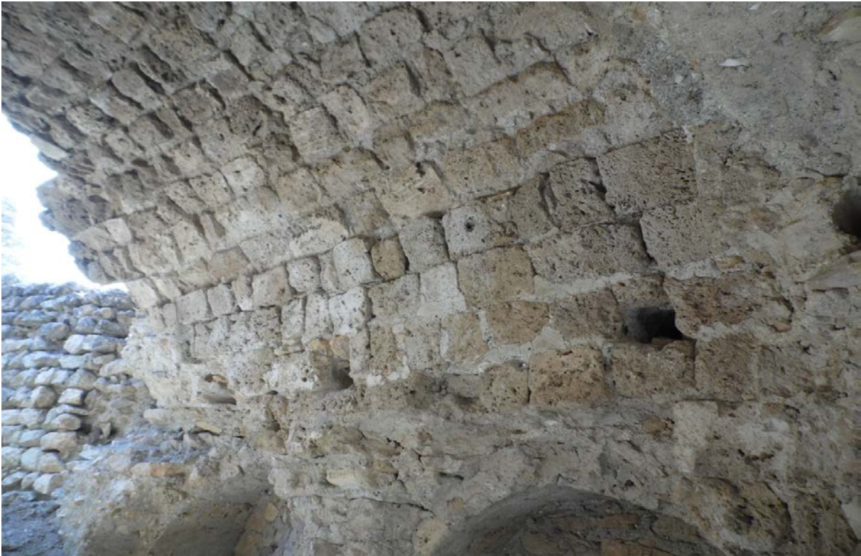
Photo 21 . North Wall (Section 6-6) and Stone Vault
