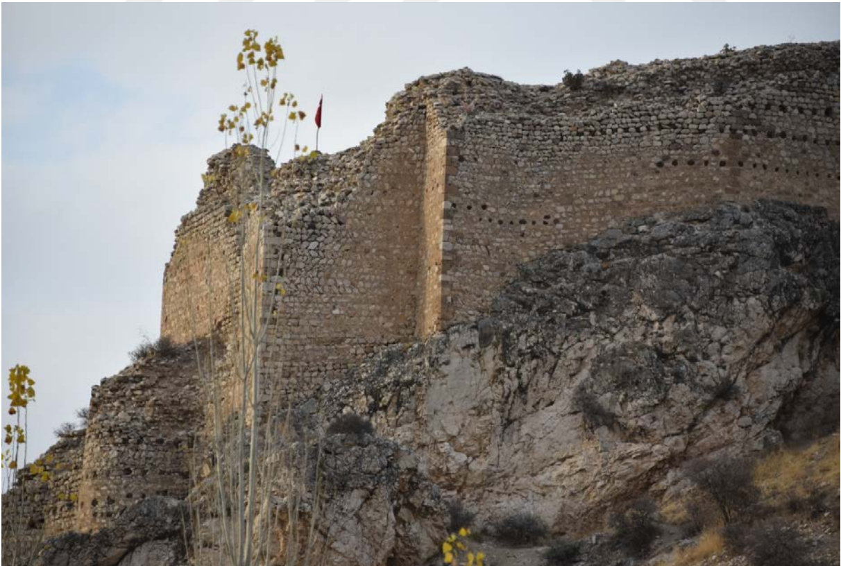
Photo 91 . Wall of GD 15-16-17-18-19
