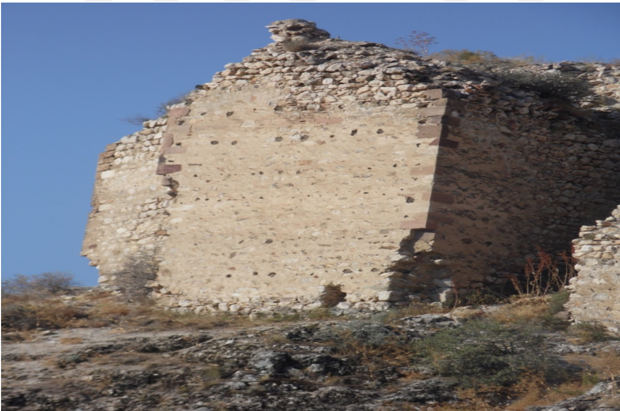
Photo 72 . Wall of DD 12-13
