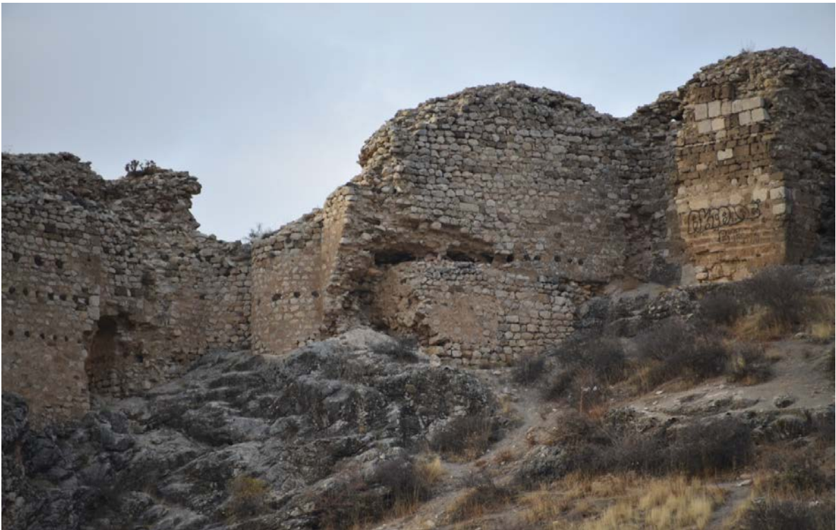
Photo 83 . Wall of GD 5-7-8-9-10-11-12
