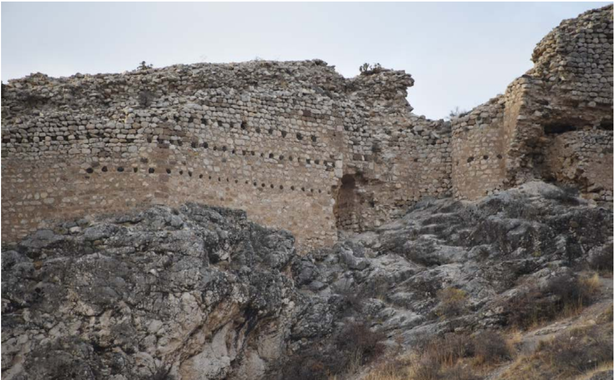
Photo 87 . Wall of GD 9-10-11-12-15-16
