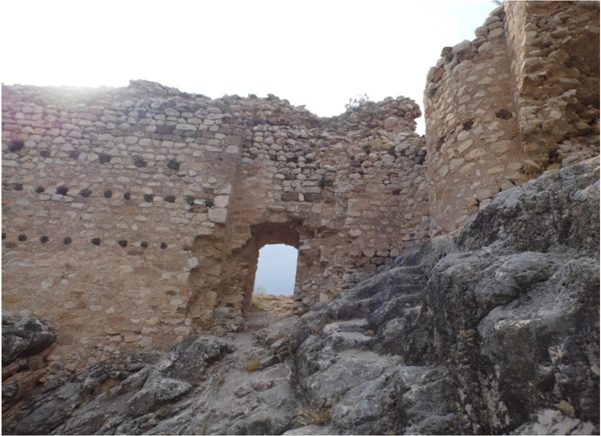
Photo 86 . Wall of GD 12 - 15
