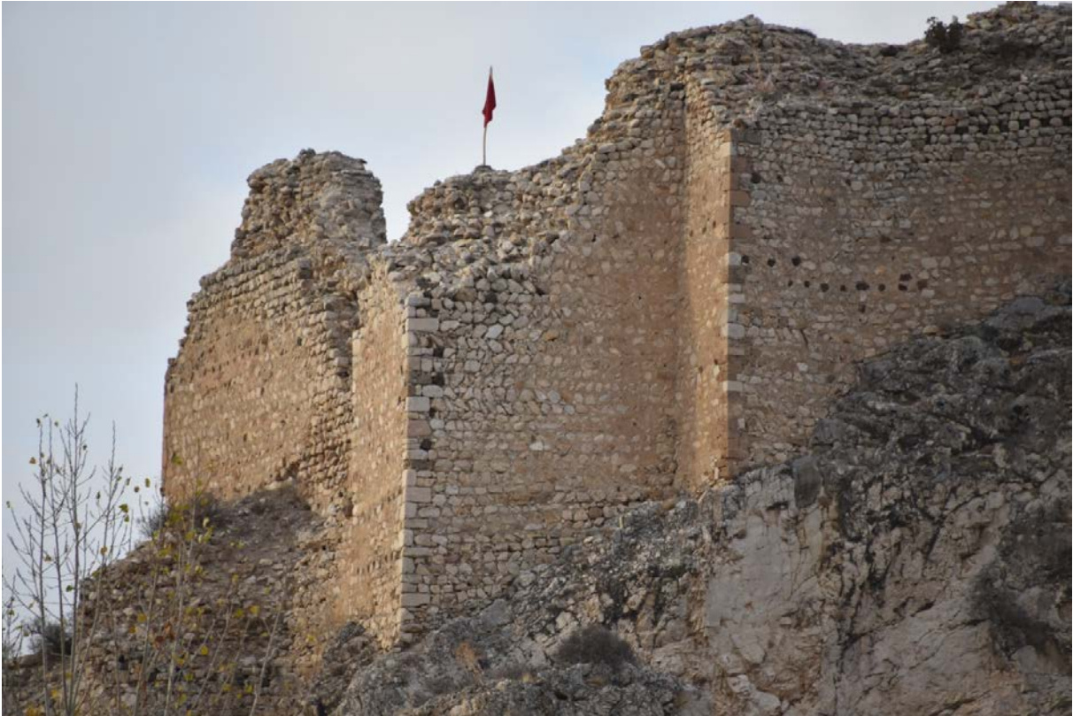
Photo 90 . Wall of GD 18-19
