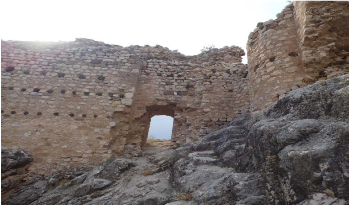
Photo 10 . Wall of GD 12-15
