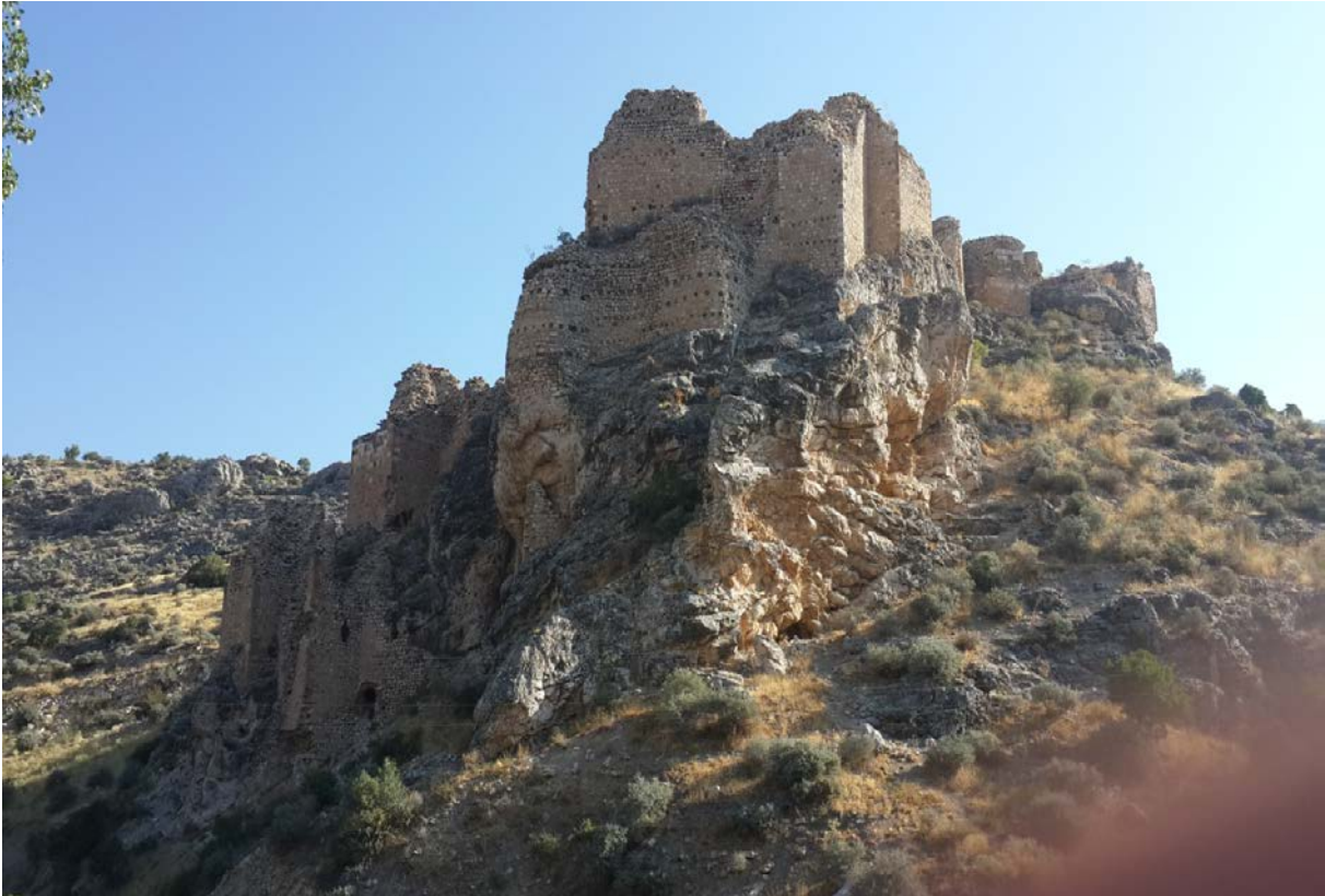
Photo 15 . South View of the Western Front
