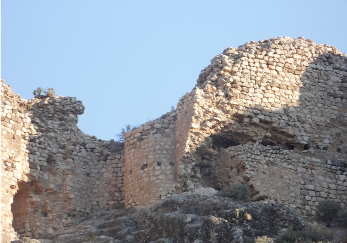
Photo 84 . Wall of GD 8-9-10-11-12
