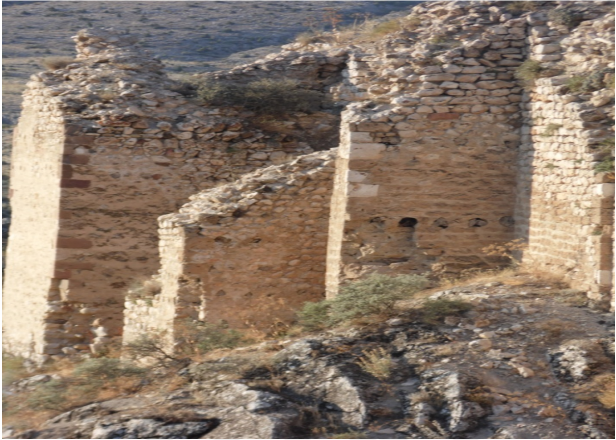
Photo 67 . Wall of DD 4-8-12
