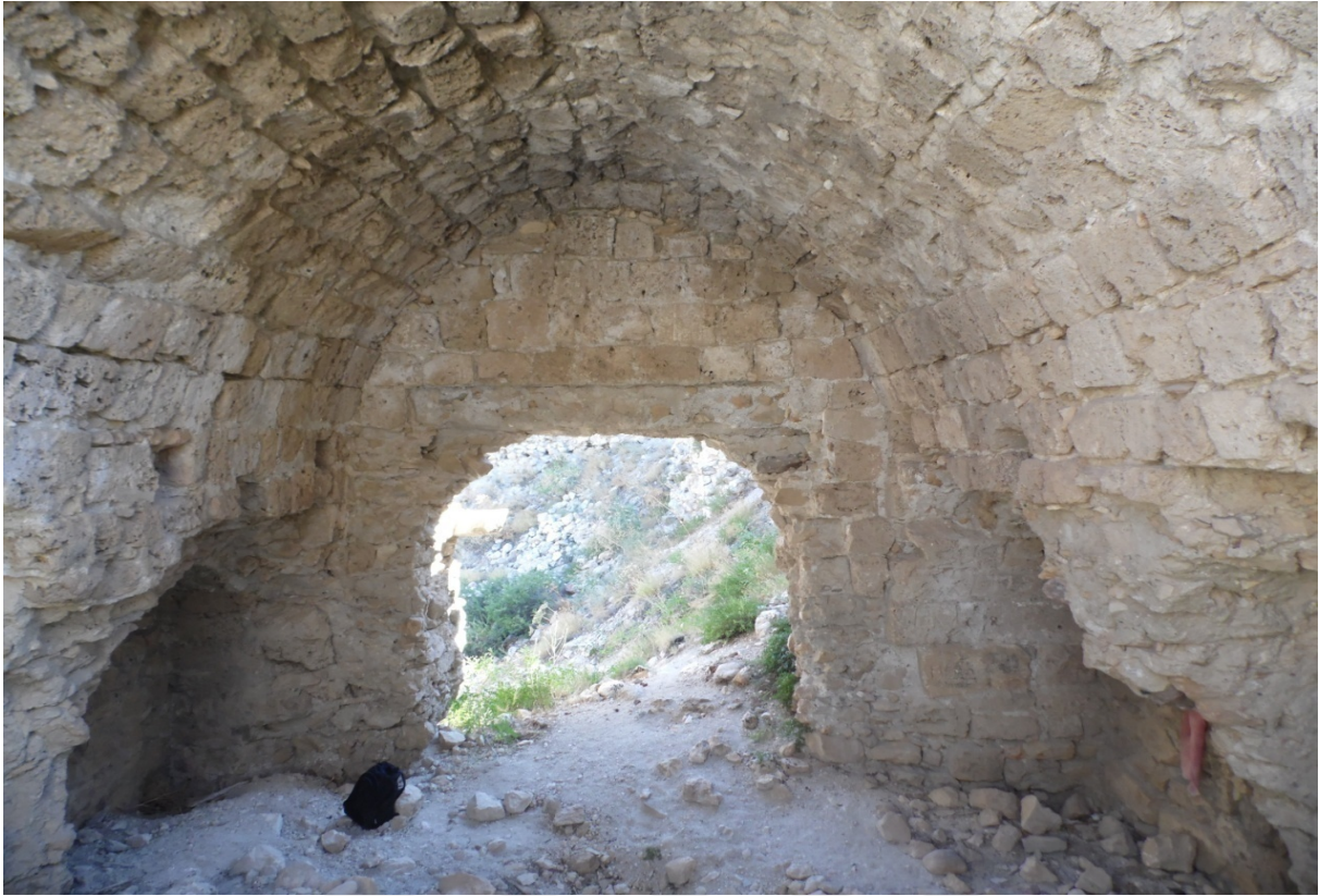
Photo 24 . Tower Eastern Wall (Section 7-7)
