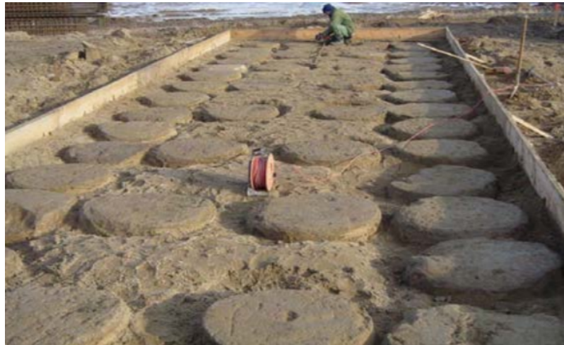
Figure 2.16: Foundation for A2 motorway bridge near Katowice (Nozu, 2005)
