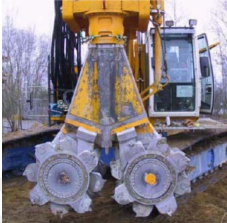
Figure 2.7: Bauer cutter soil mixing (Fiorotto et al., 2005)
