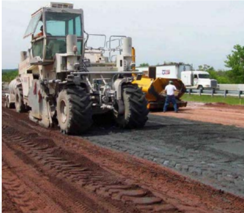
Figure 2.2: A road reclaimer mixes soil with moist conditioned fly ash (Beeghly, 2003).
