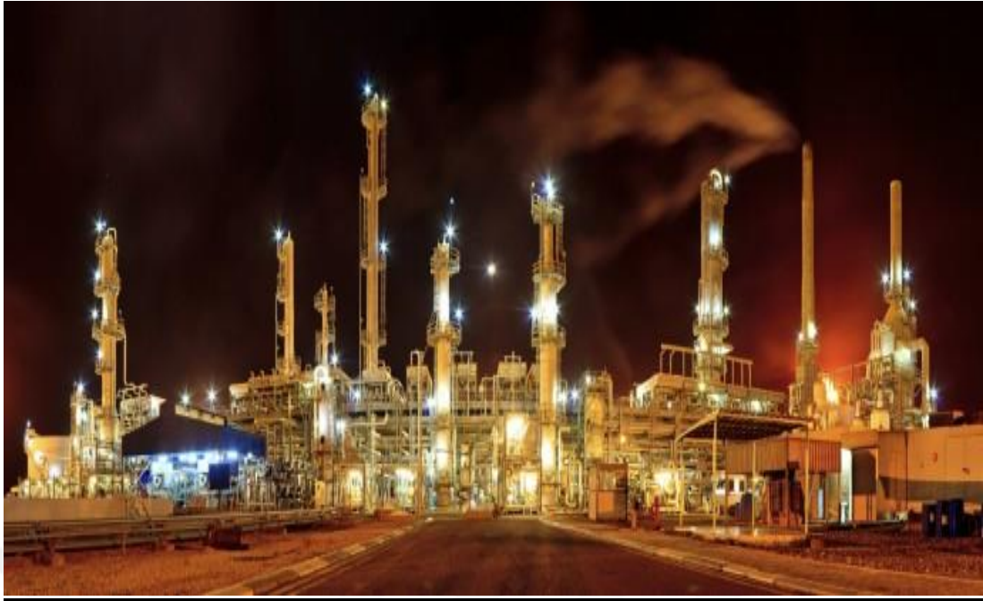
Figure 4.3 Night view of Kawergosk refinery.
