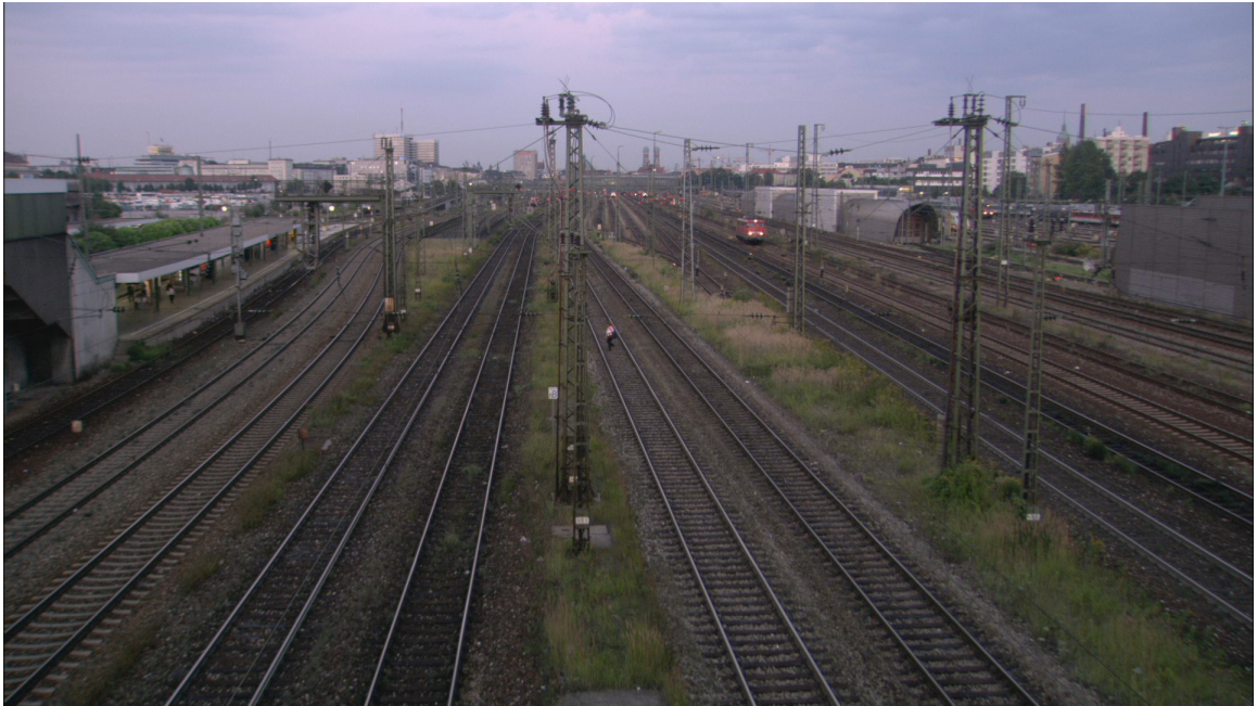
Figure 24: A frame from the video segment Station2.
