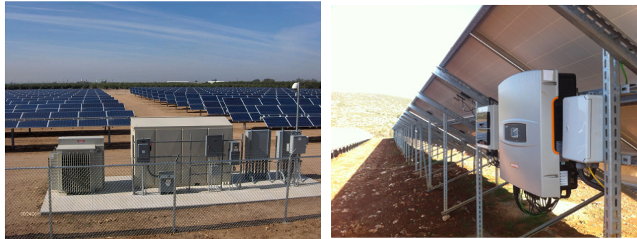
Figure 2-21 Placement of Central Inverters and String Inverters [72]
