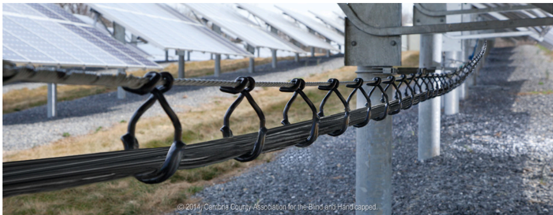
Figure 2-22 Cabling of PV Systems [73]
