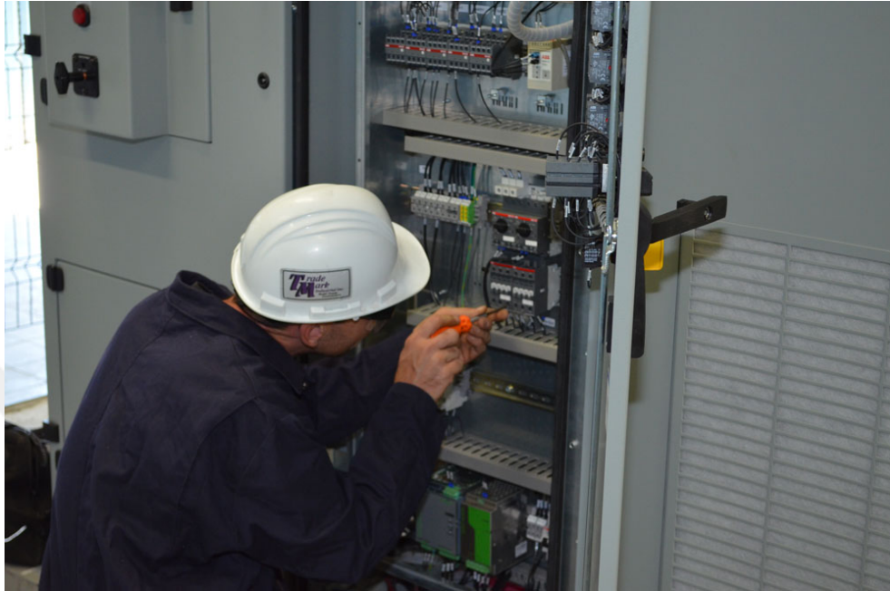
Figure 2-23 Installation of Main Electricity Distribution Board [74]
