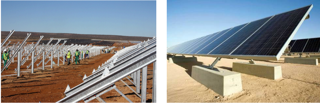
Figure 2-20 Horizontal Metal Bars and PV Modules Installation [71]
