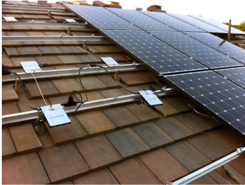
Figure 2-6 Micro Inverter Installation under each PV Modules [46]
