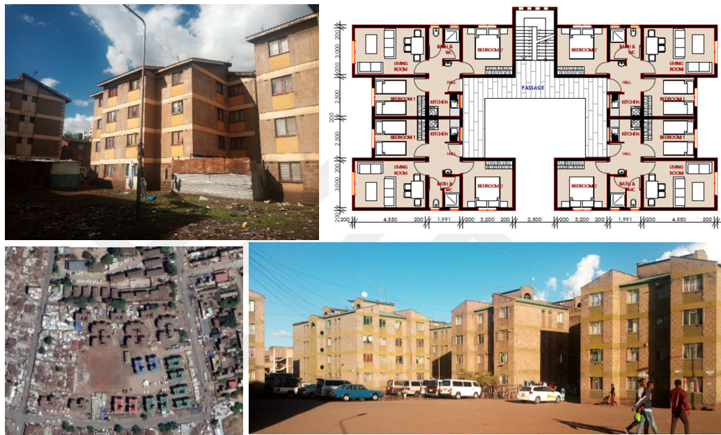
Figures 3.11, 3.12, 3.13, and 3.14: Photos, floor layout and site layout of a two bedroom block in KENSUP Soweto East
