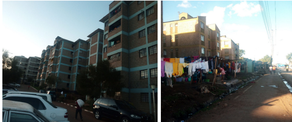
Figure 4.53 and 4.54: Public spaces in KENSUP Soweto are visible from all units thus encouraging security however Pumwani’s layout lacks a boundary wall to demarcate it from the street and nearby informal settlements hence compromises security
