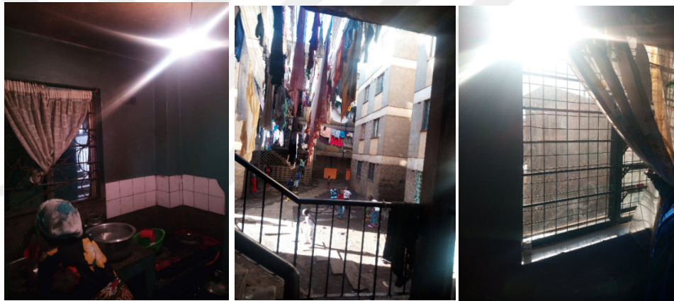
Figure 4.37, 4.38 & 4.39: Interior spaces especially in Pumwani were poorly lit in addition to obstruction from drying laundry
