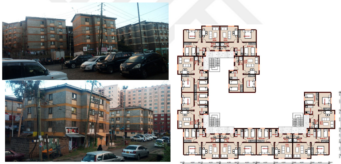
Figures 3.2, 3.3, 3.4, 3.5 and 3.6: Photos, floor layout and site layout of a two bedroom block in Kibera Nyayo highrise
