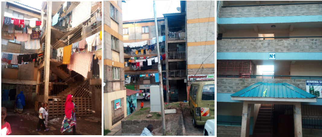
Figure 4.21, 4.22 and 4.23: Access staircases for Pumwani, Nyayo highrise and Soweto East respectively
