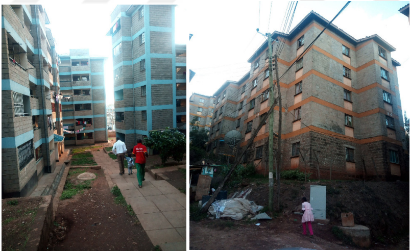
Figure 4.25 and 4.26: Lack of ramps within the landscape of Soweto East and Nyayo highrise despite the steep topography
