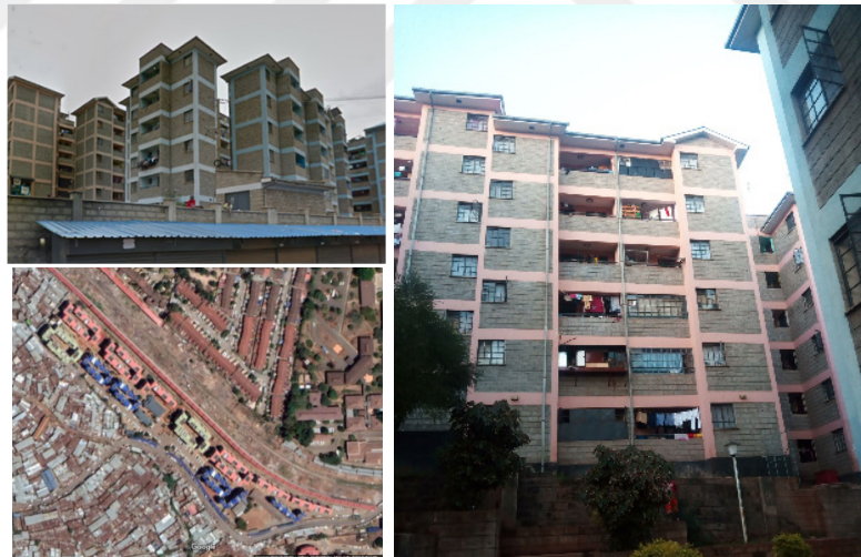
Figures 3.7, 3.8, 3.9, and 3.10: Photos, floor layout and site layout of a two bedroom block in KENSUP Soweto East
