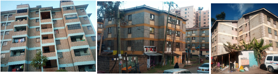
Figure 4.29, 4.30 and 4.31: Conversions added onto housing in KENSUP Soweto East, Nyayo highrise and Pumwani respectively
