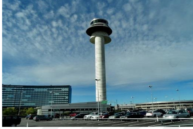
Şekil 2.17. Arlanda airport control tower, Stockholm, Sweden
