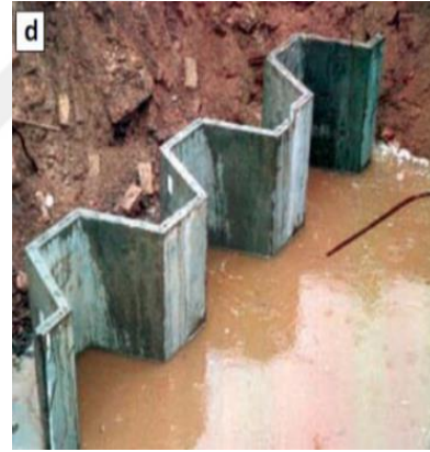
Installed Sheet Piles
