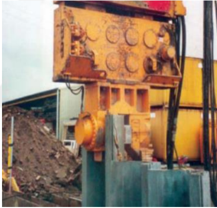
Hammered UYPB sheet piles
